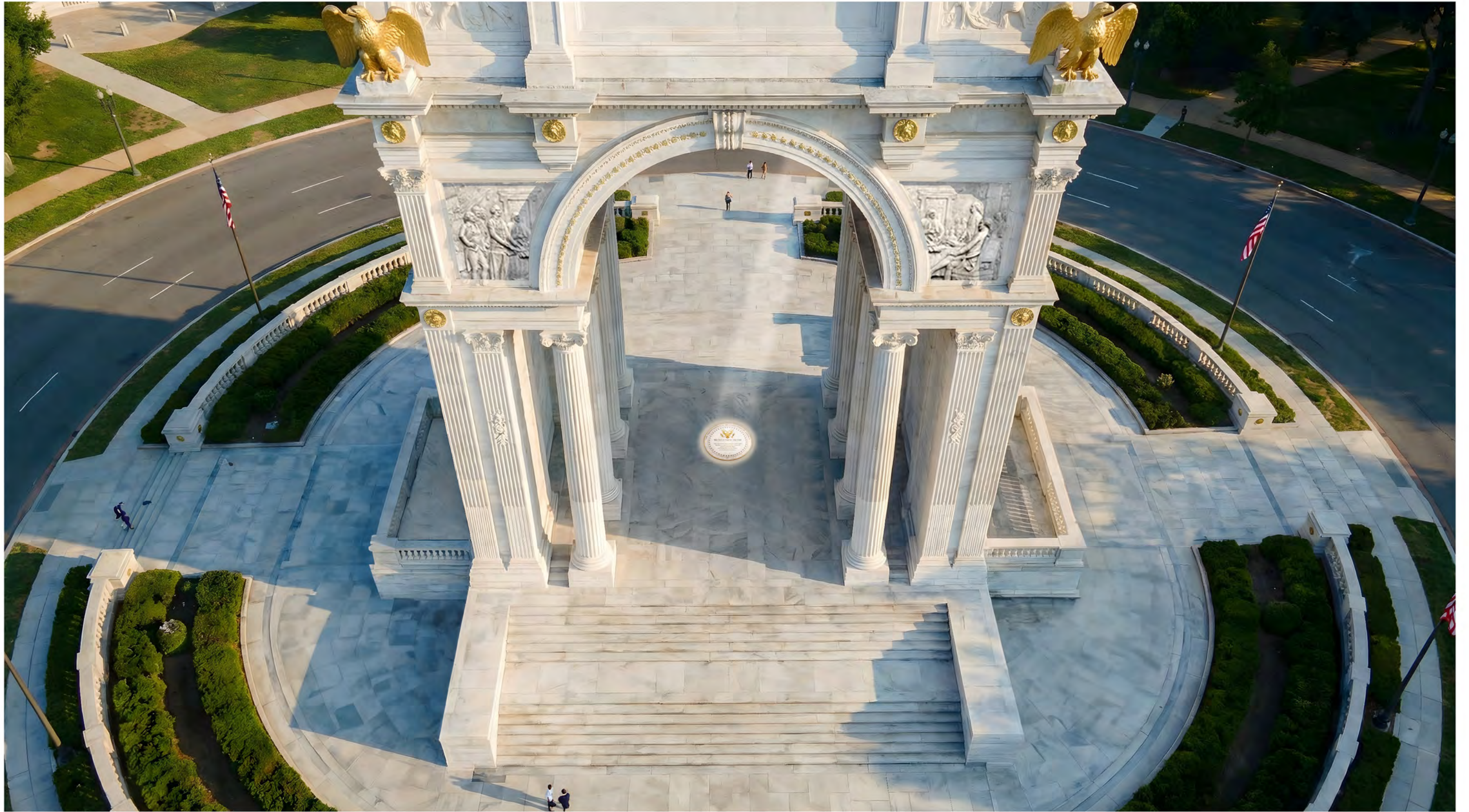
Aerial Perspective Showing Sunbeam Reaching the Floor Through the Arch Roof and Illuminating the Stone Datum Within the Arch Shadow
