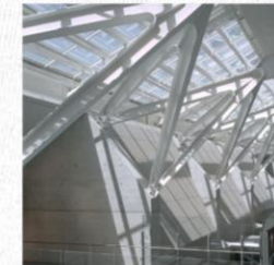
BUILT-UP STEEL STRUCTURE
