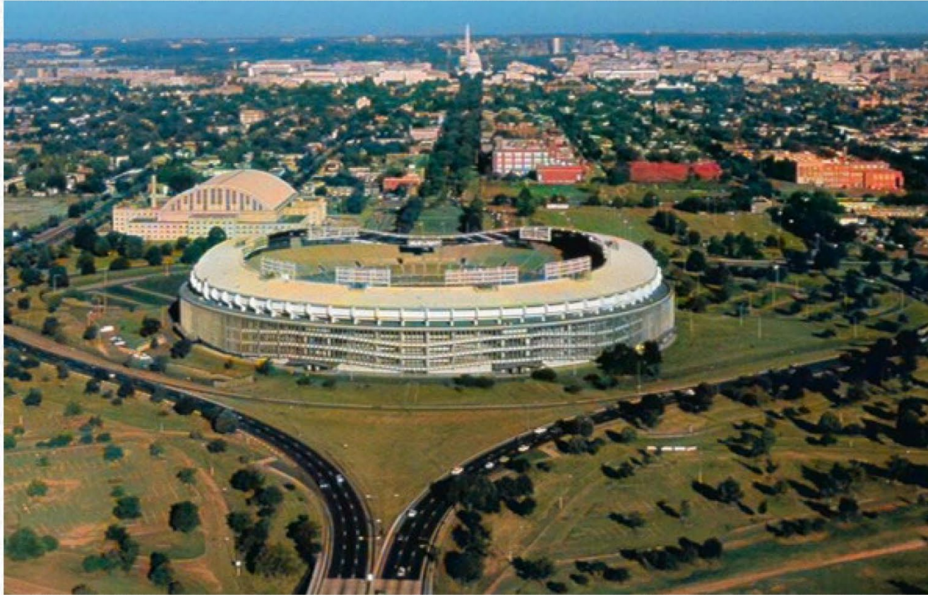
View of RFK Stadium looking west toward the U.S. Capitol Building.
