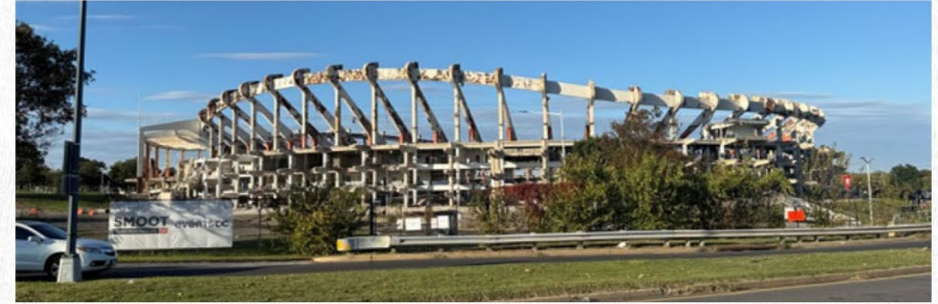
Demolition of RFK Stadium as of Fall 2025, from Independence Avenue Southeast.
