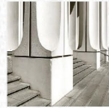
C.I.P. CONCRETE STRUCTURE
