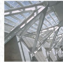
BUILT-UP STEEL STRUCTURE
