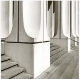
C.I.P. CONCRETE STRUCTURE
