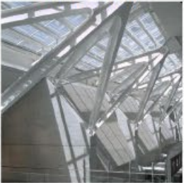
BUILT-UP STEEL STRUCTURE
