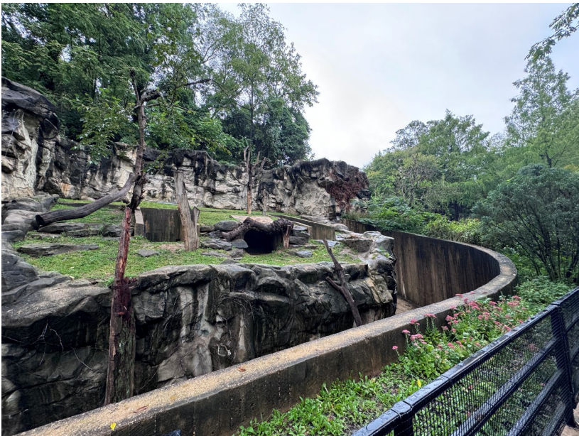
VIEW 2 (looking east): West Habitat Yard - shows signs of deteriorating rockwork, dead trees, and the moat condition
