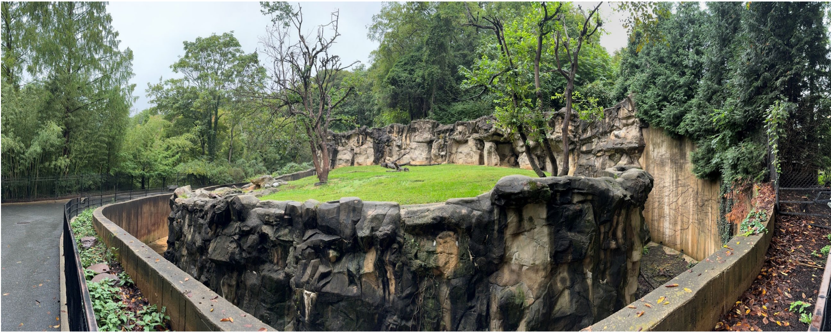
VIEW 1 (looking west): East Habitat Yard East habitat yard shows signs of deteriorating rockwork, dead trees, and the moat condition
