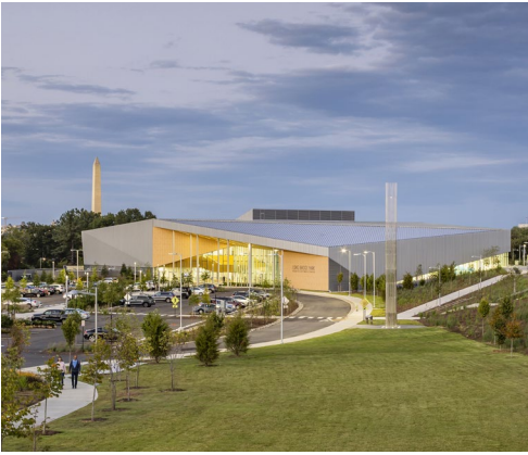
Long Bridge Aquatics and Fitness Center
