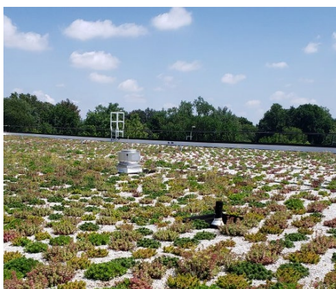
PSOC Vegetated Roof
