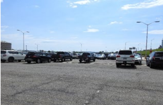
Rehabilitate Deteriorated Pavement in South Parking Lot
