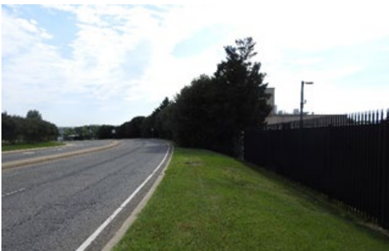
Install Missing Sidewalk Section
