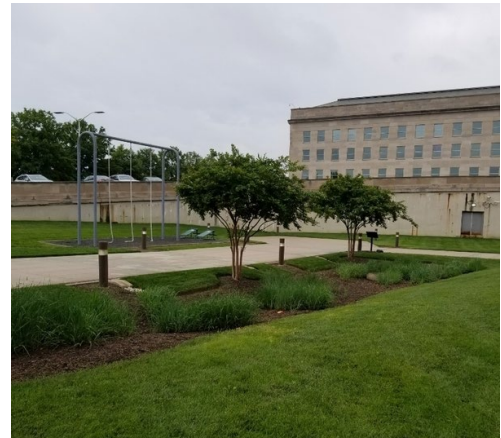
PAC Entrance Existing Bioretention Area
