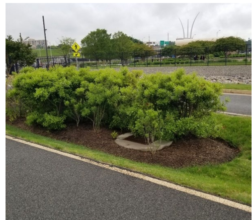
Corridor 5 VACP Existing Bioretention Area
