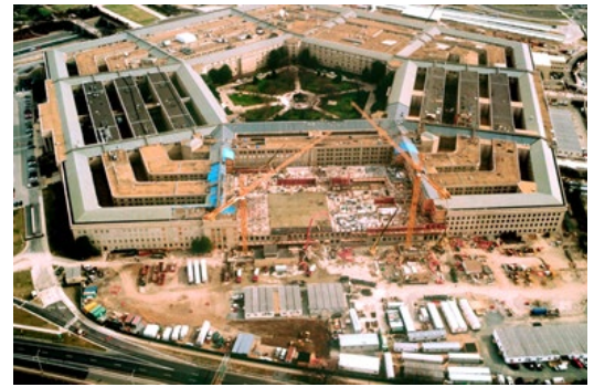
Sections of E, D, and C Rings Removed from West Side for Reconstruction after 9/11 Terrorist Attack, February 6, 2002
