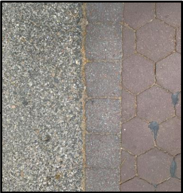
Existing asphalt tie-in to hexagonal pavers with border course.
