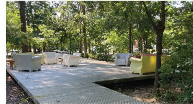
The metal decking would offer a permeable surface that would enable the retention of trees.
