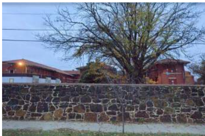
H Historic Campus Stone Wall
