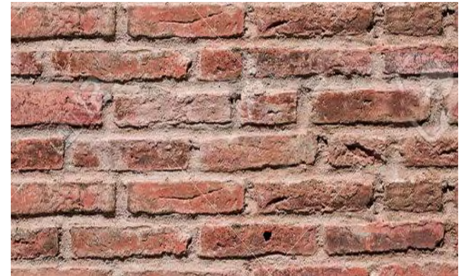
Existing Brick - To Be Restored and Repointed
