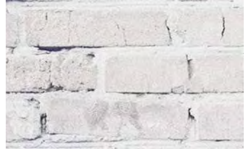
Existing Brick - Repointed, Restored, Repainted
