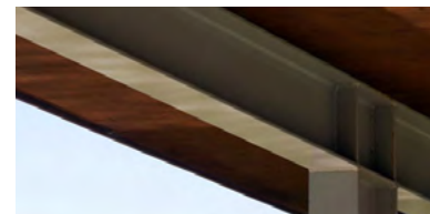
Architectural Exposed Structural Steel
