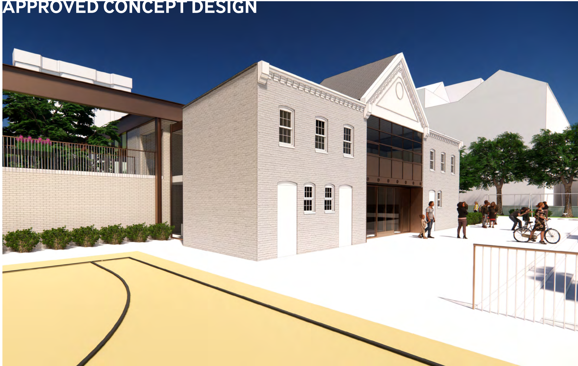
Existing Brick - Repointed, Restored, Repainted
