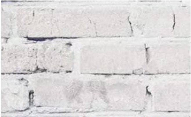
Existing Brick - Repointed, Restored, Repainted
