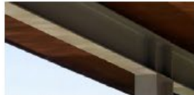
Architectural Exposed Structural Steel
