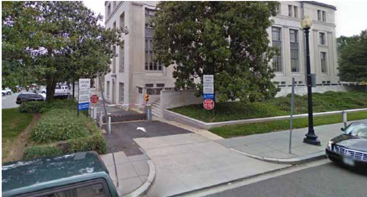
FRB-East | Vehicular Entrance at 20th St NW
