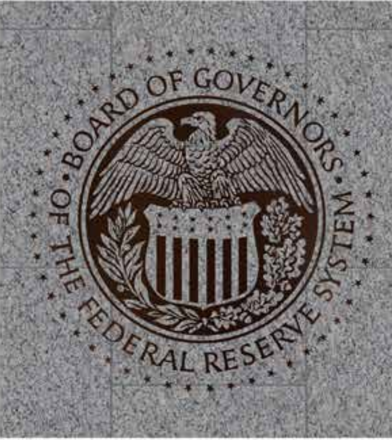
Figure 3-61: Paver Seal Detail Seal Fabricated Entirely From Dark Bronze Metal Inlaid Into Stone Pavers
