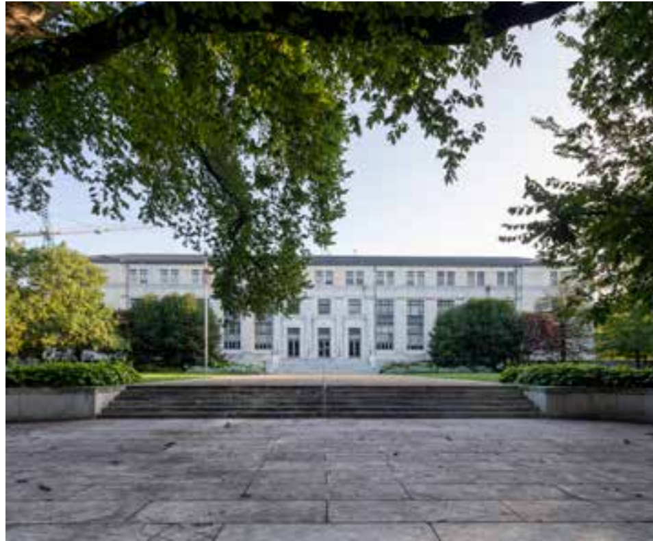
13. FRB-East Building South Facade
