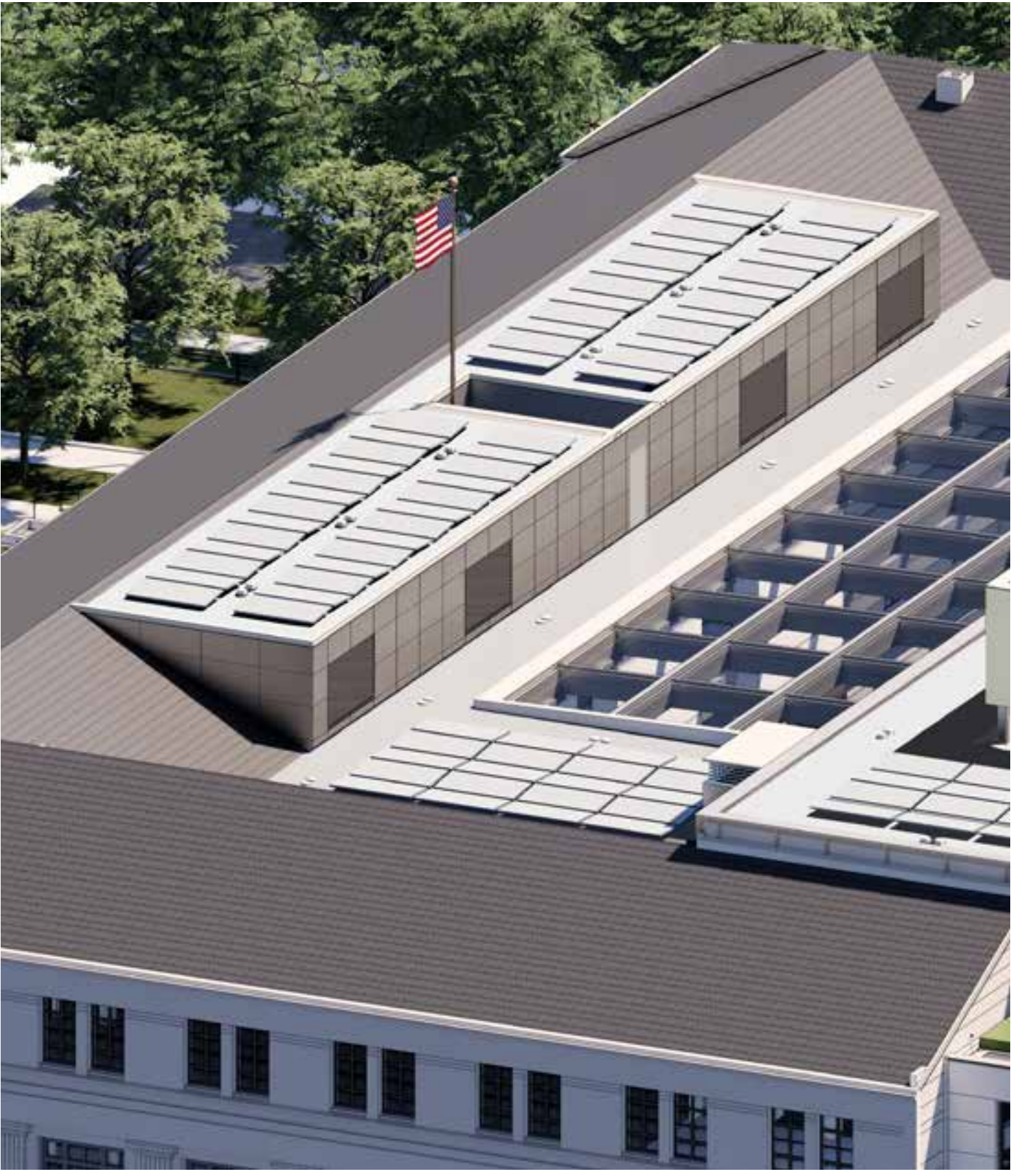
Figure 3-17: Expanded and Modernized Mechanical Penthouse on FRB-East Building
