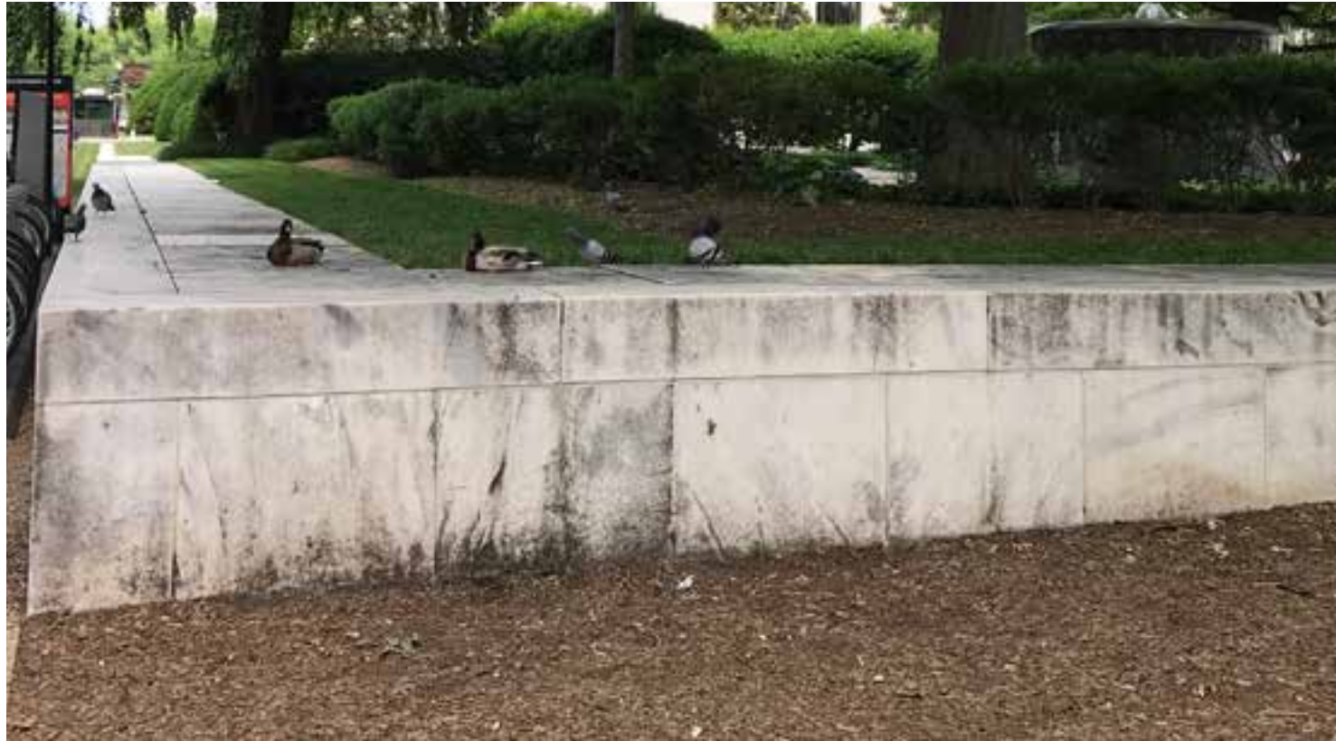
Existing Site Retaining Wall as a Barrier
