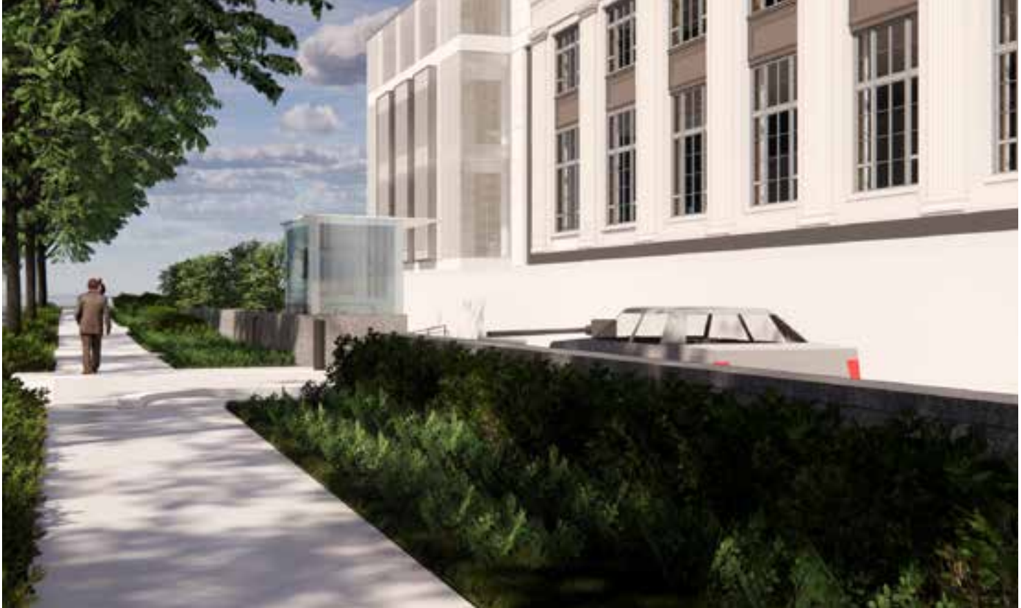
Figure 3-46: View of FRB-East south lawn officer's post from south
