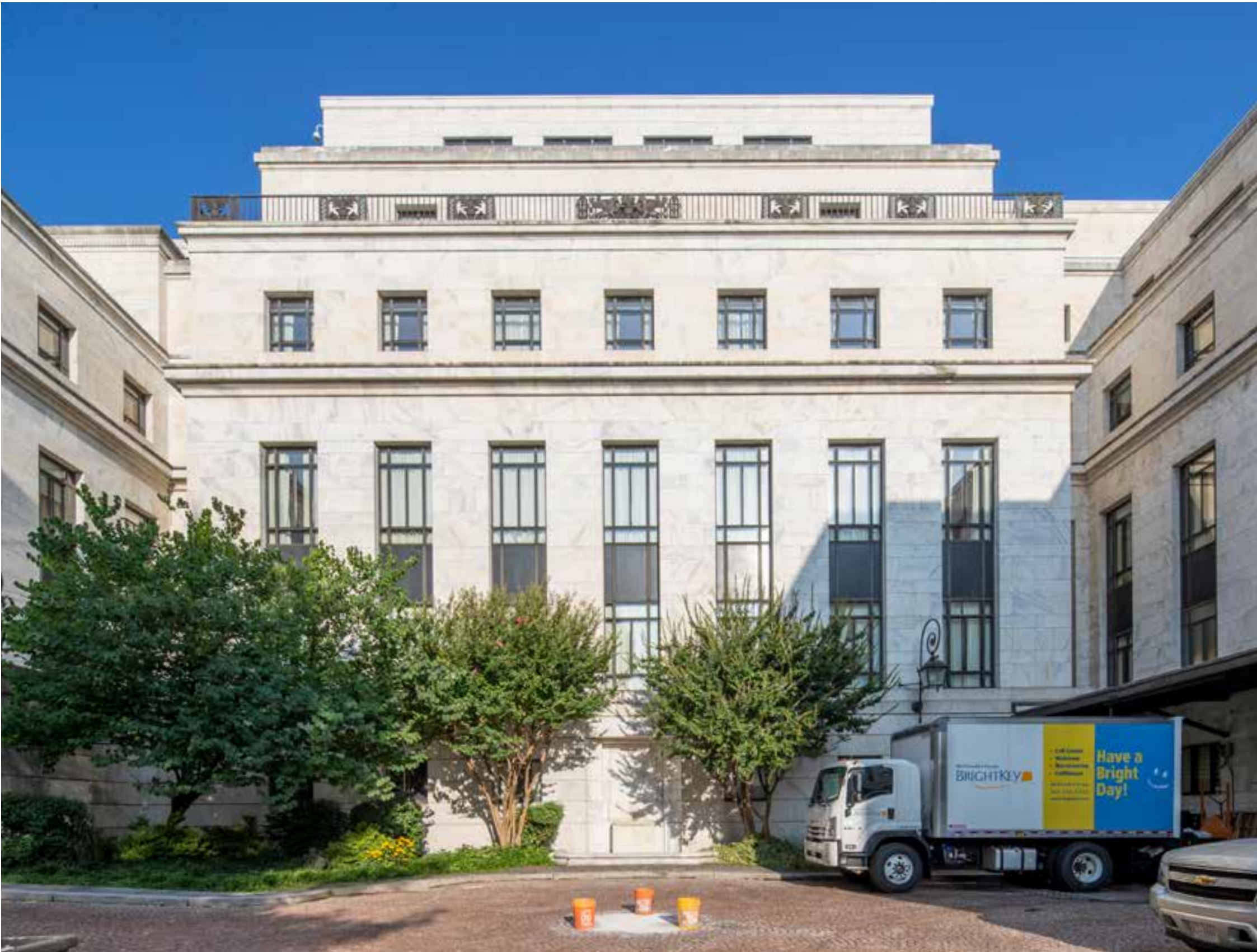
Figure 3-3: Double height bronze windows with Alberene stone spandrel panels
