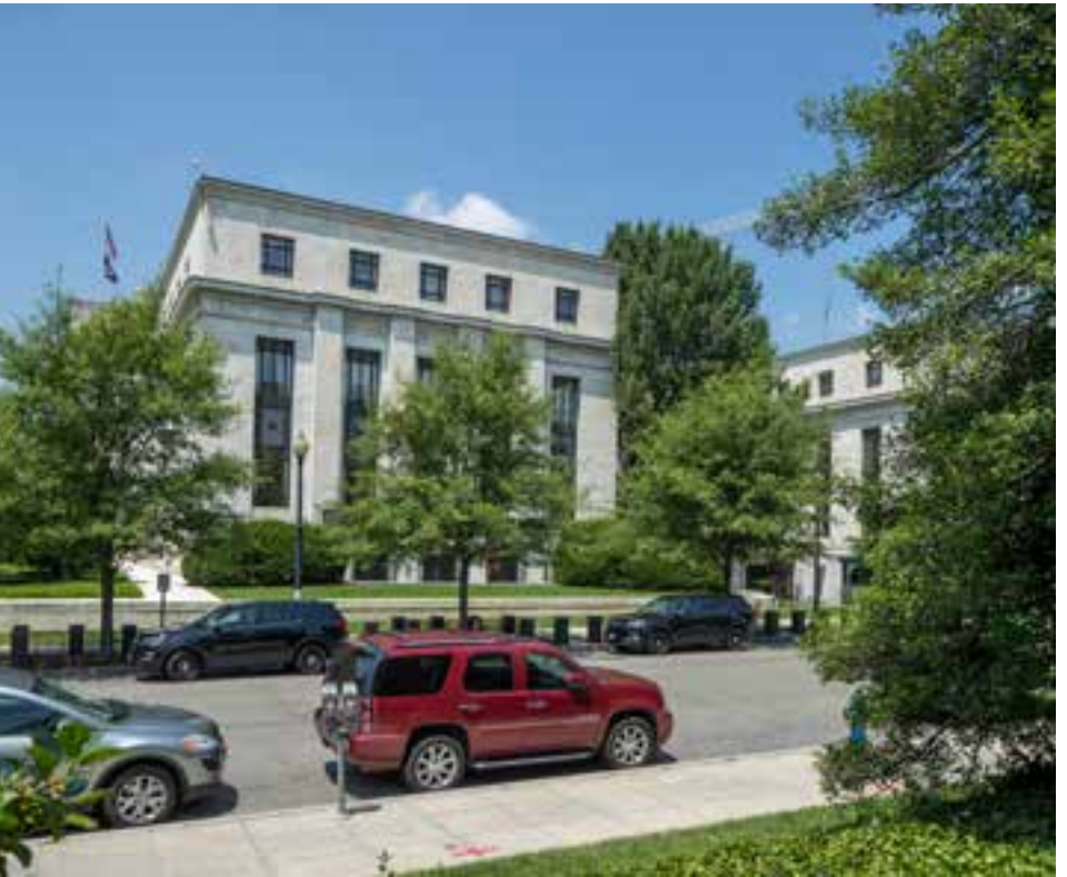
3. Eccles Building East Facade
