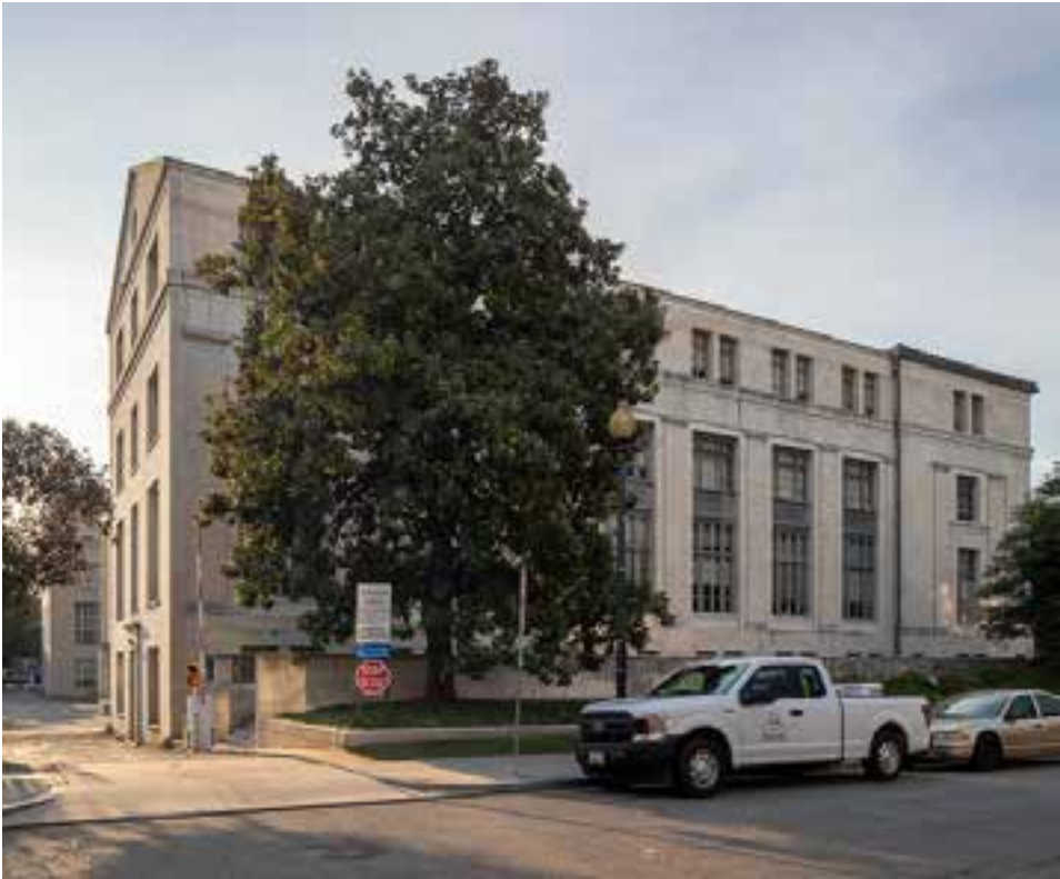
9. FRB-East Building West Facade
