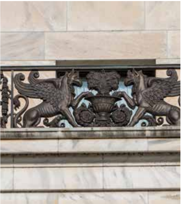
Figure 3-4: Bronze railing detail
