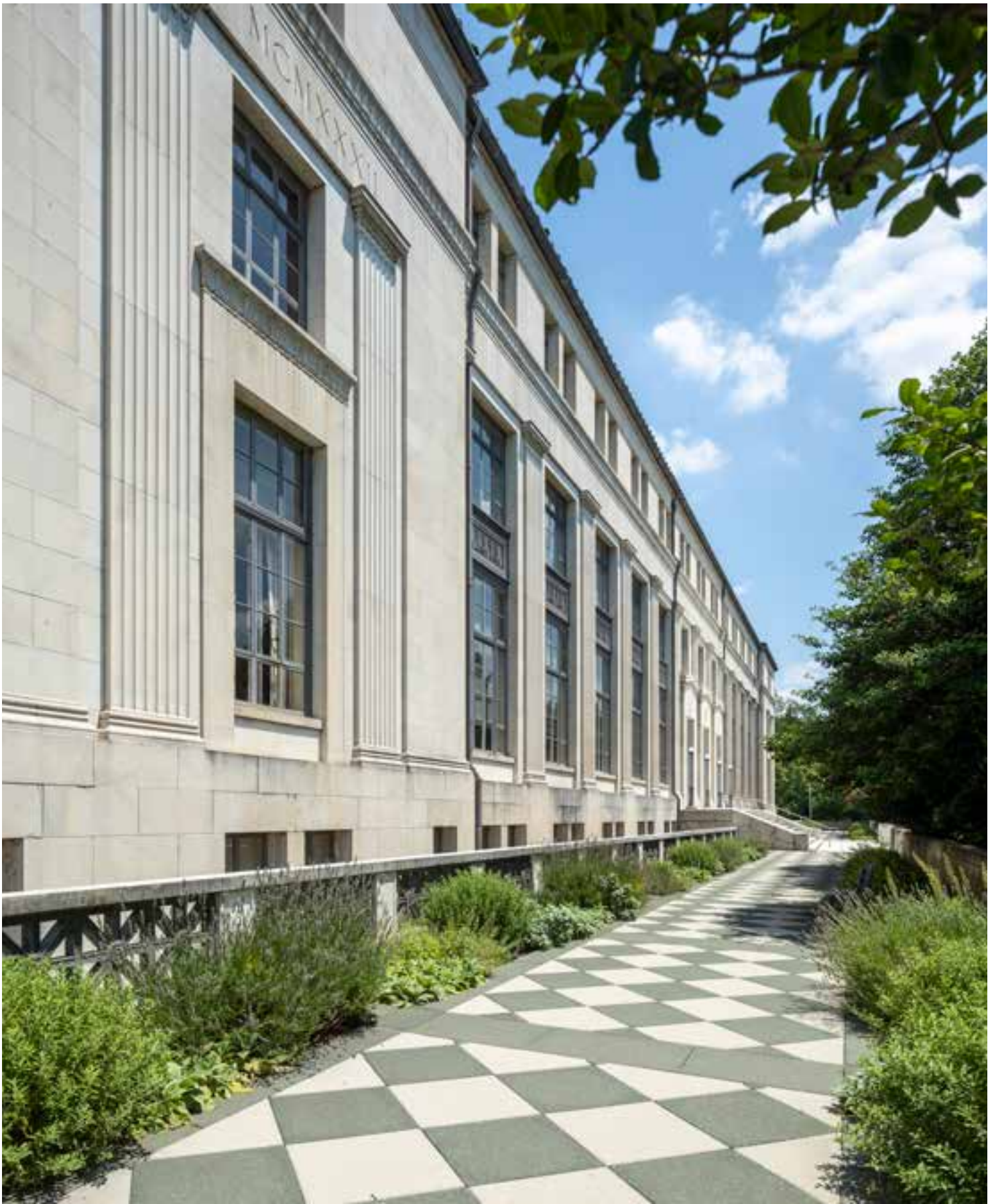
Figure 3-1: FRB-East Building South Facade and Terrace
