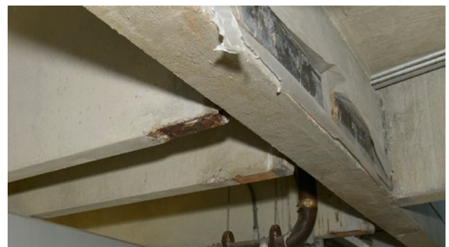
Missing Concrete in the NSF Suitland Parking Garage Source: Department of Navy
