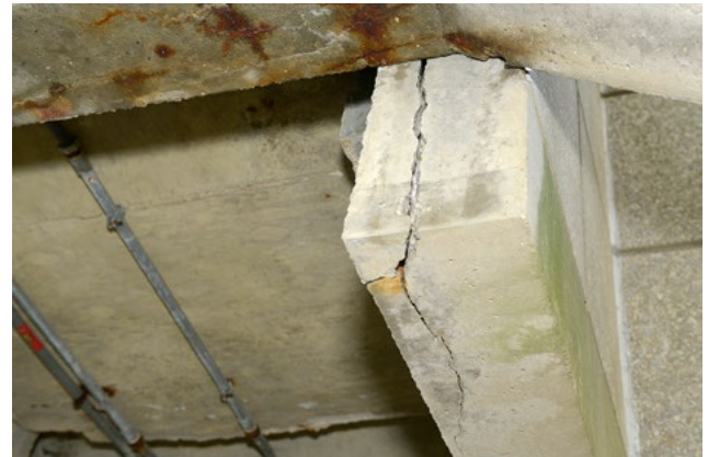
Deterioration of Parking Garage at NSF Suitland Source: Department of Navy
