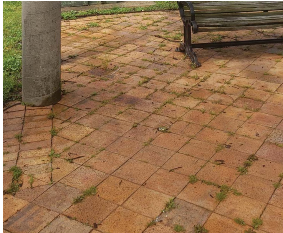
SQUARE PAVER, DIAMOND BOND AMPHITHEATER PLATFORM AND ENTRY BATHROOM AREA
