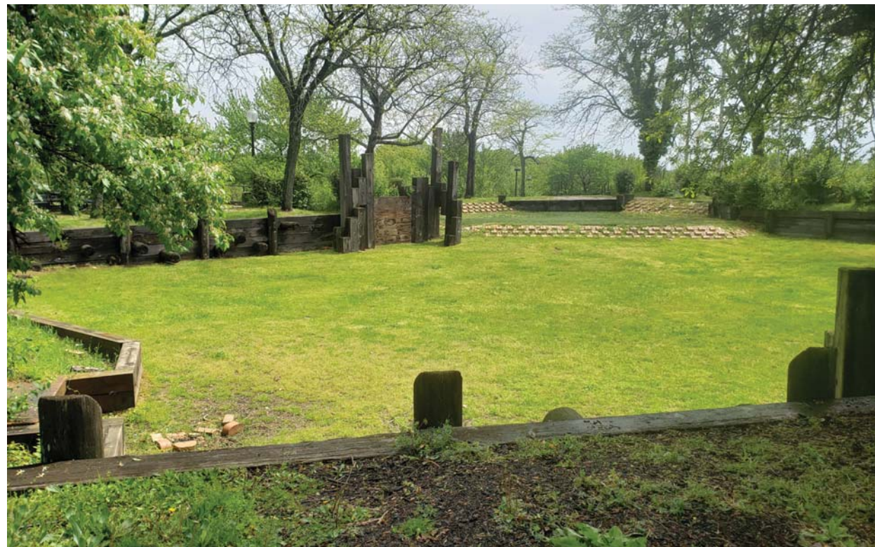
RAILROAD TIE WALLS
