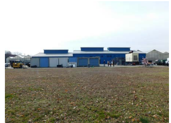
Area North of Existing SG Headhouse
