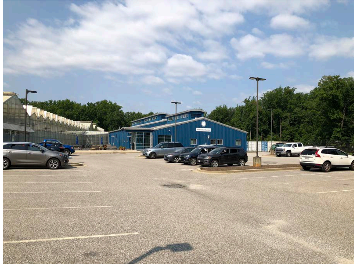
Existing SI Gardens Parking Lot and Headhouse
