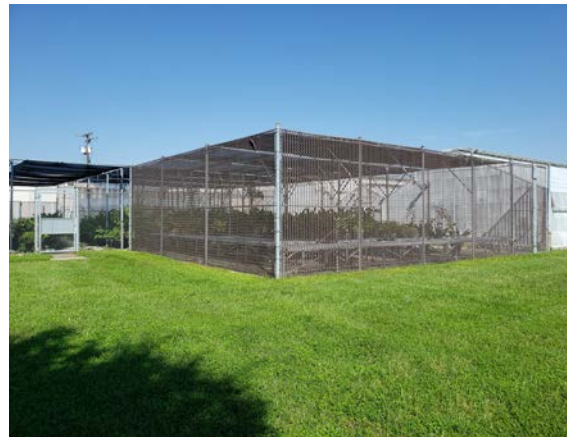
Existing Botany Shade Structure
