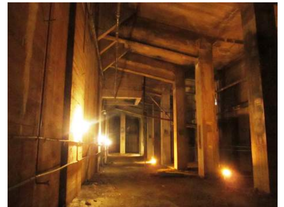
6 - VIEW OF THE RAISED TERRACE UNDERCROFT
