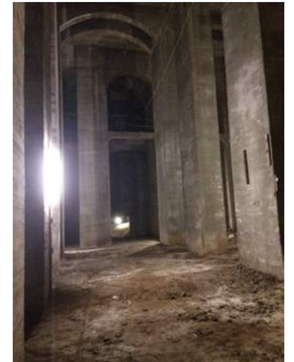
4 - VIEW OF THE CHAMBER UNDERCROFT
