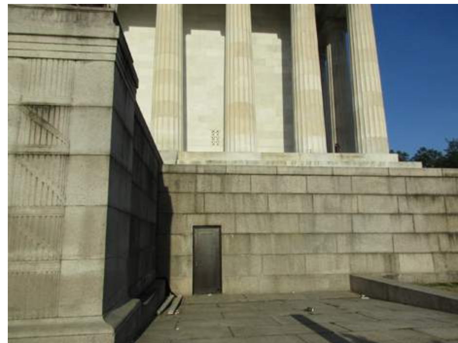
4 - SOUTH-EAST UNDERCROFT DOOR
