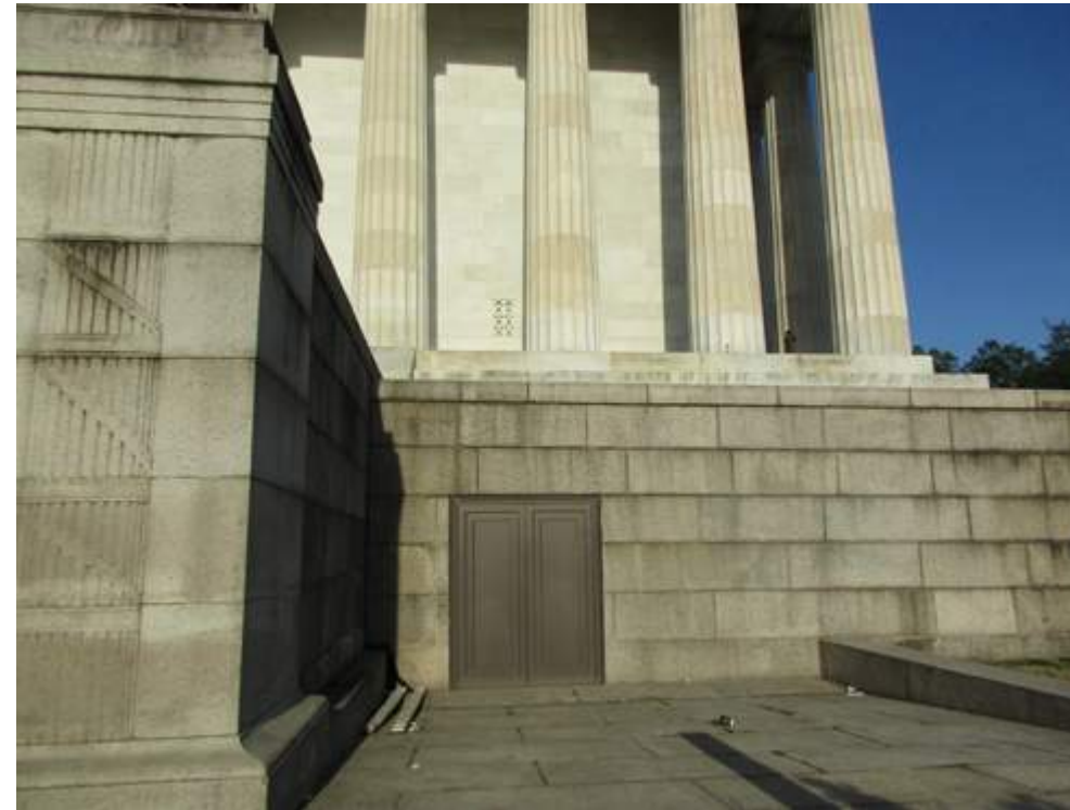
2 - NORTH-EAST UNDERCROFT GATES
