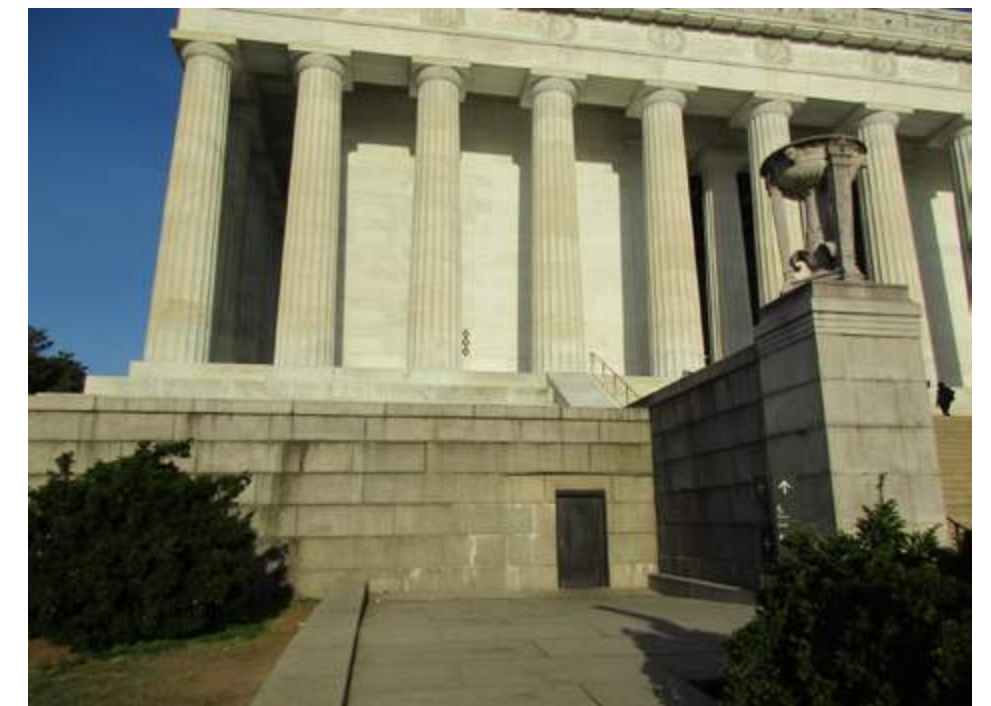
5 - NORTH-EAST UNDERCROFT DOOR
