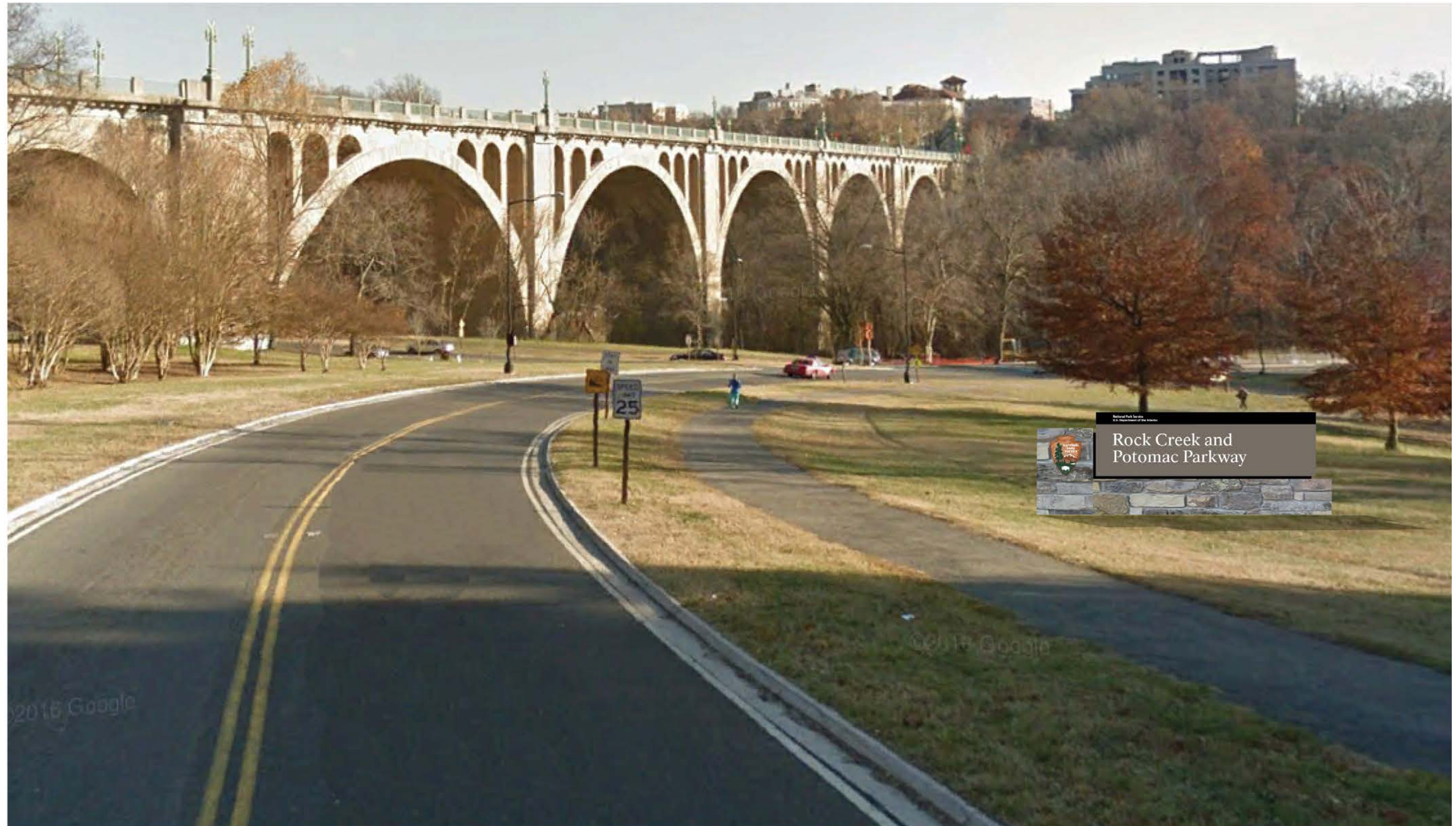
Rock Creek and Potomac Parkway looking southbound in the vicinity of Calvert Street, NW
