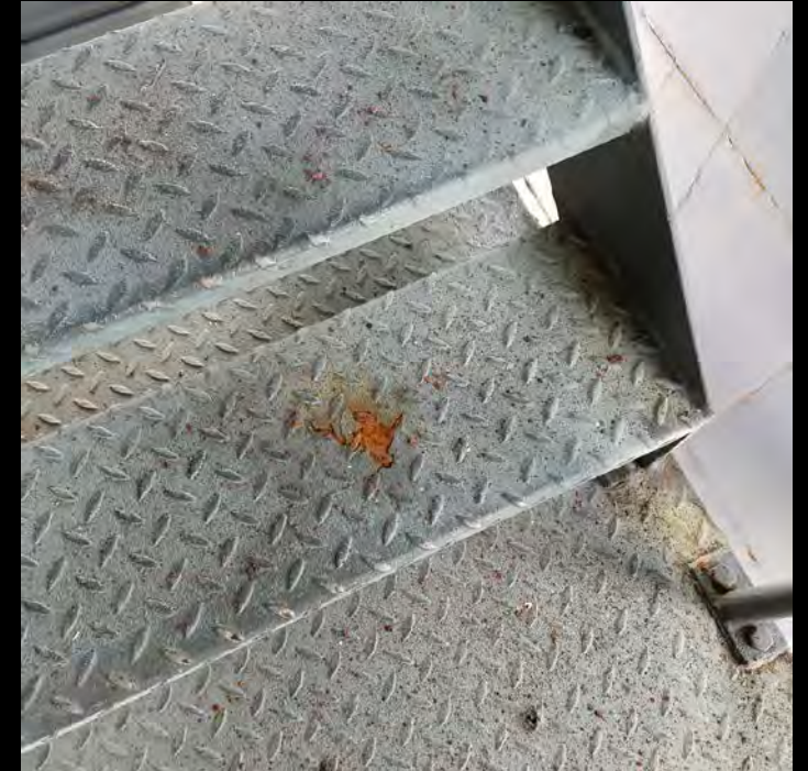
LANDING AND TREAD REPLACEMENT
