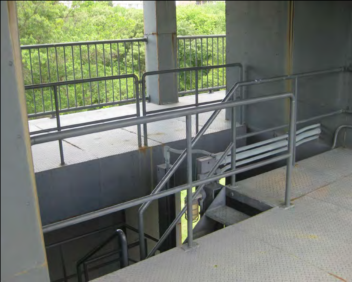
EXISTING STAIR CONFIGURATION AT OBSERVATION DECK 1
