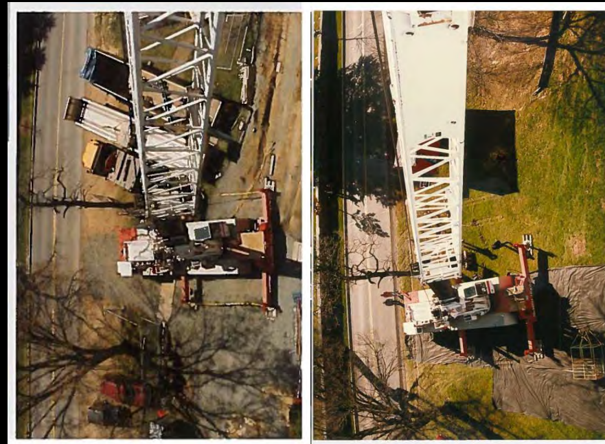
1995 Construction staging along N. Marshall Drive
