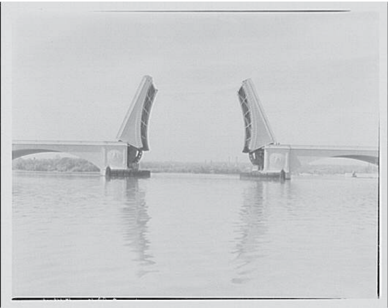
An undated photograph of the bascule span in the open position. Credit: Library of Congress
