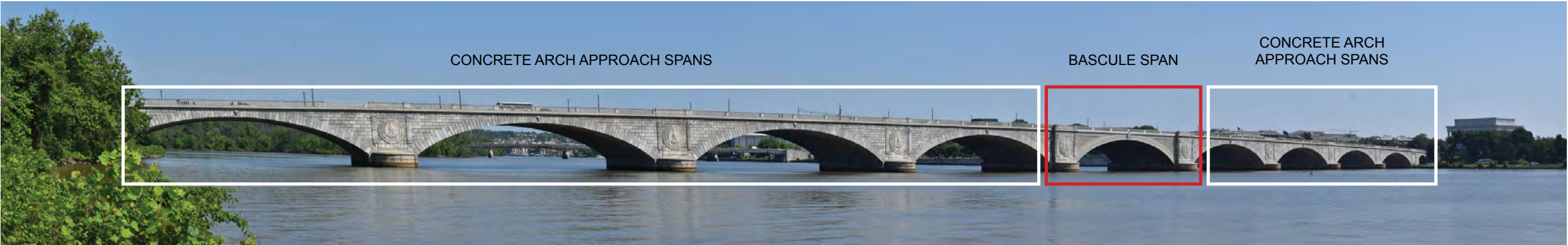
South Elevation looking North. Credit: Nathan Holth, courtesy HistoricBridges.org
