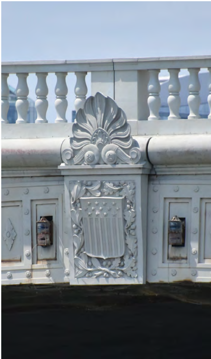
A cast aluminum cartouche sits at the center of the bascule span, flanked by red and green navigator lights Credit: Nathan Holth, courtesy HistoricBridges.org
