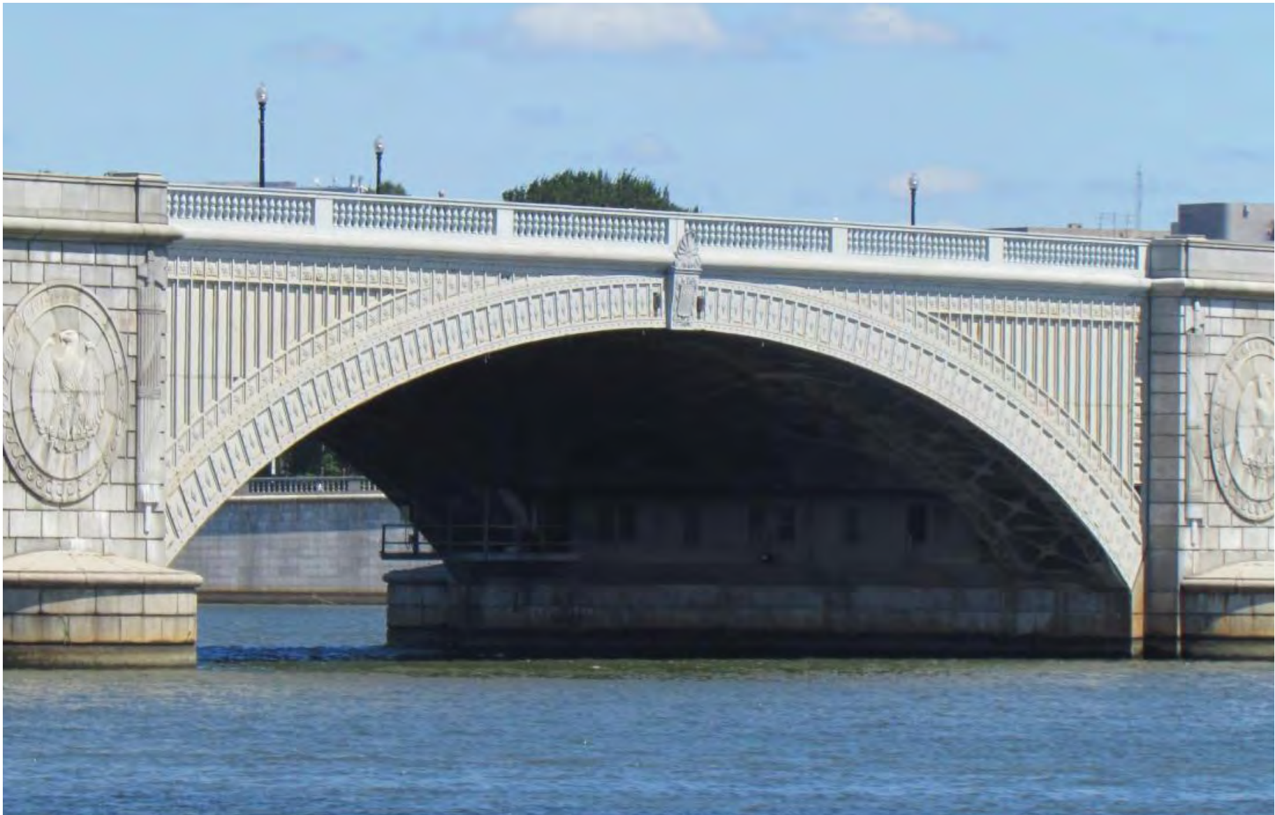
The bascule trusses on both sides are faced with ornamental steel fascia panels with decorative cast aluminum stars and buttons Credit: Nathan Holth, courtesy HistoricBridges.org
