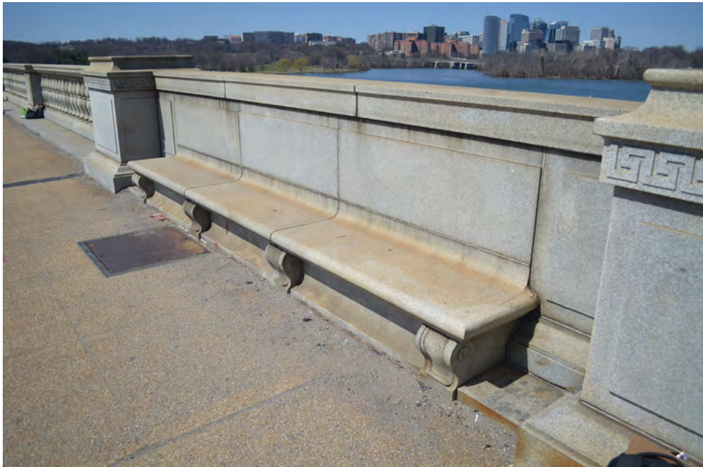
Granite bench seats. Credit: Quinn Evans Architects
