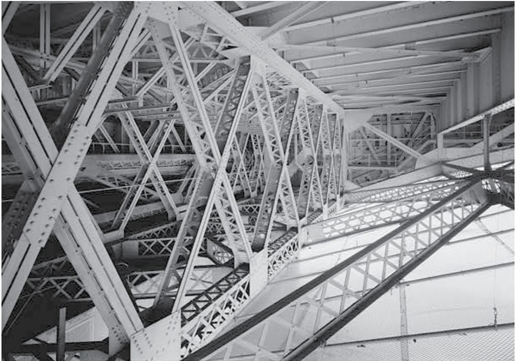
Transverse floor beams and bottom lateral bracing of the bascule span Credit: Library of Congress. Jet Lowe, Historic American Engineering Record, 1991.
