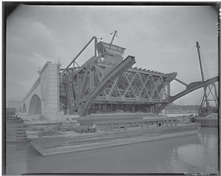
An undated photograph of the bascule span under construction Credit: Library of Congress
