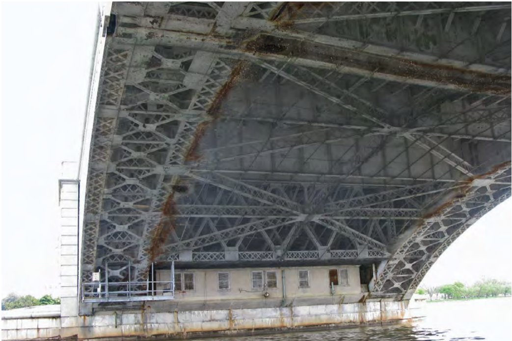
View of bascule span steel structure and west side of Abutment 2 including operating machinery room. Credit: Federal Highway Administration
