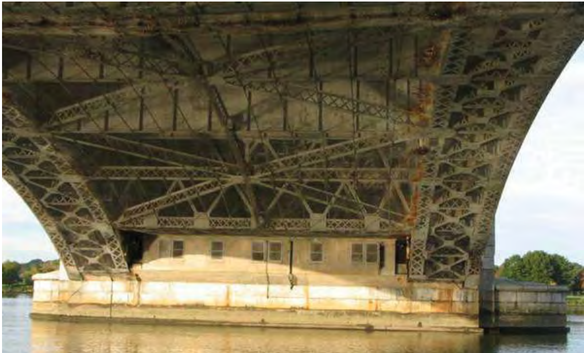
View of bascule span steel structure and east side of Abutment 3 including operating machinery room. Credit: Kiewit
