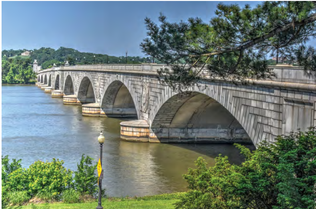
Granite facing on the concrete arch spans and cast-in-place concrete forming the underside of the approach span arches. Credit: Nathan Holth, courtesy HistoricBridges.org
