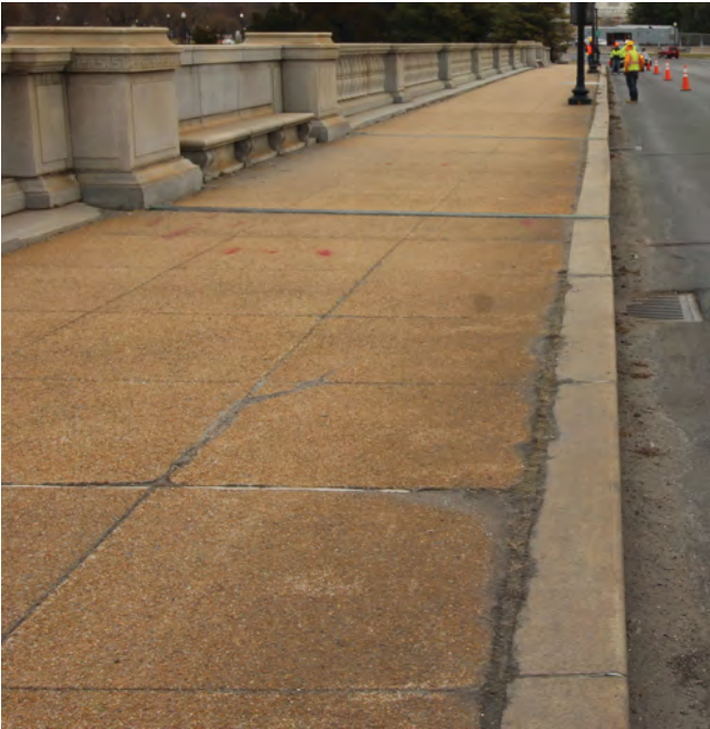
Exposed aggregate sidewalk and granite curbing Credit: Quinn Evans Architects
