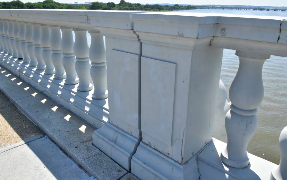
Aluminum balustrade. Credit: Quinn Evans Architects
