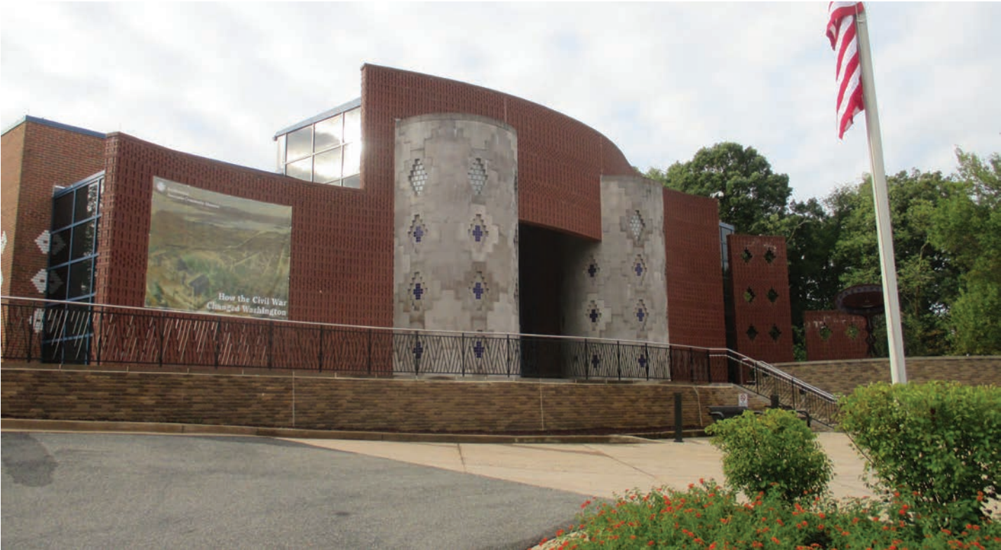
EXISTING BUILDING FACADE & LANDSCAPE MATERIALS
