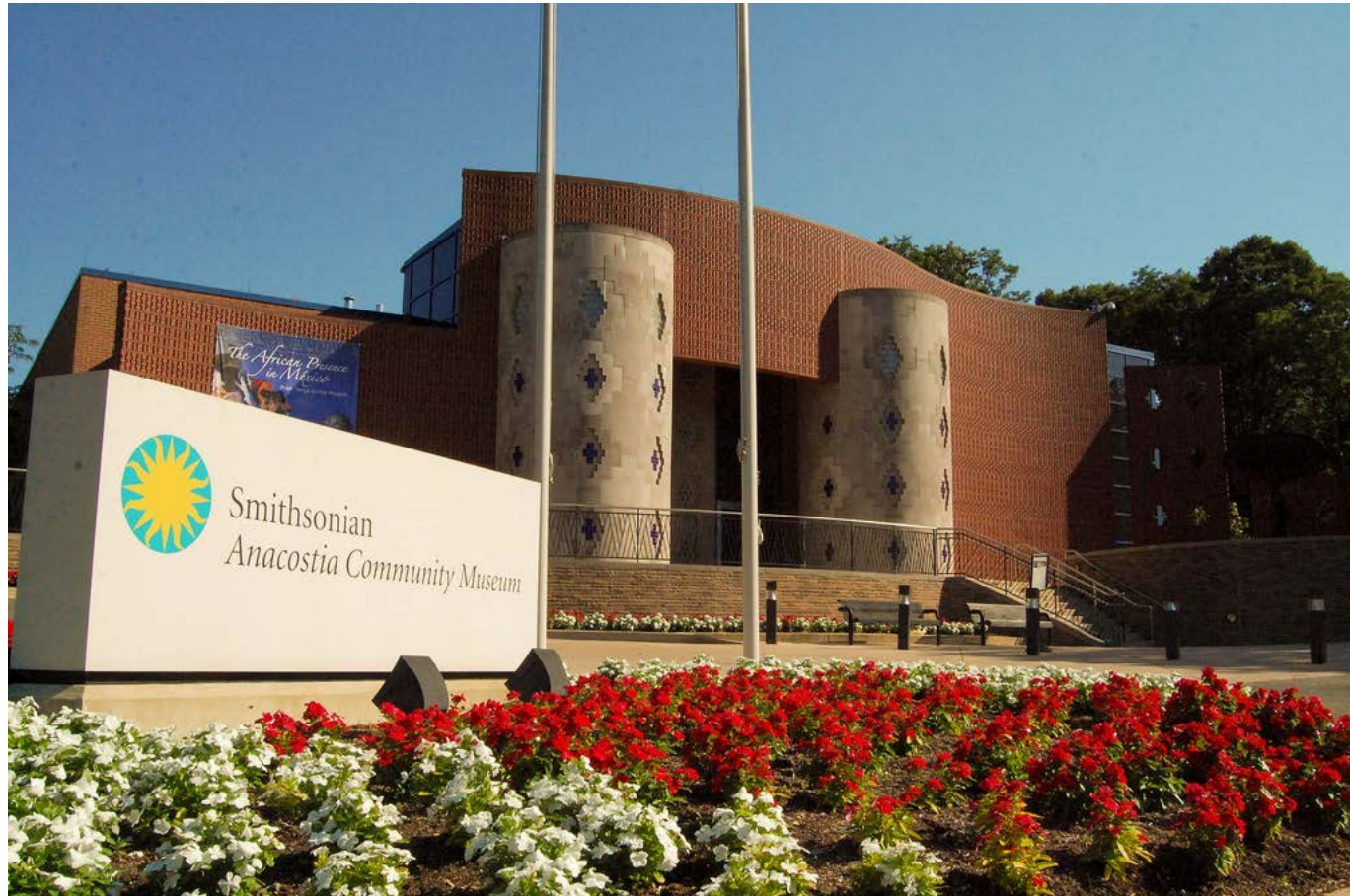
VISITORS' ENTRANCE: VIEW SOUTHEAST FROM MAIN ENTRANCE
