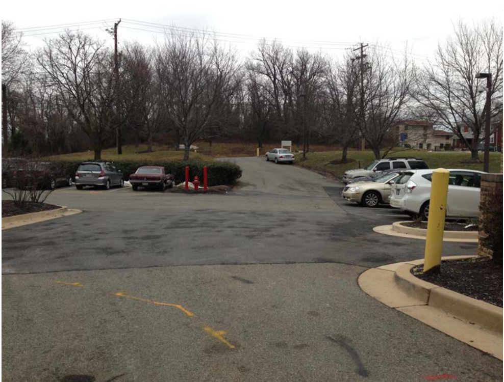
PARKING AREA: VIEW NORTH TOWARD EXIT
