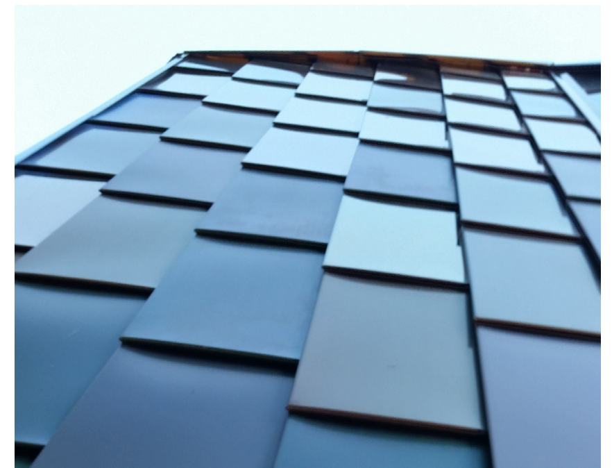
Metal Panel - Flat Lock Installation
