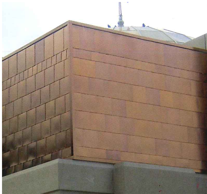
Metal Panel - Flat Lock Installation
