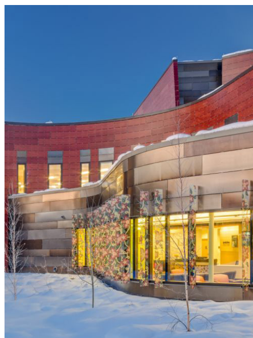
Metal Panel - Flush Joint
