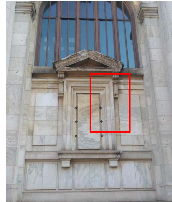
Anchor points in grout joints
