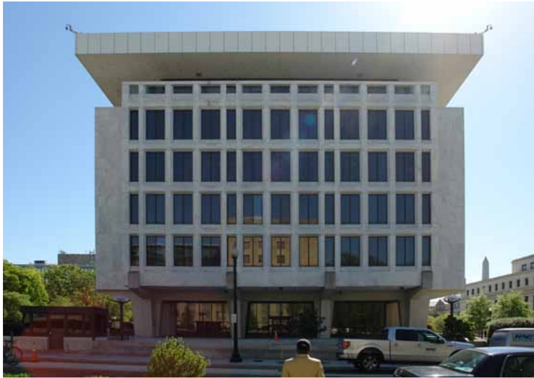
7 WEST ELEVATION VIEW
