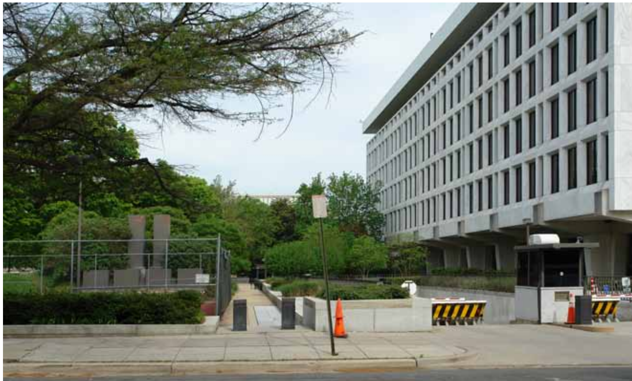
9 NORTHWEST CORNER VIEW
