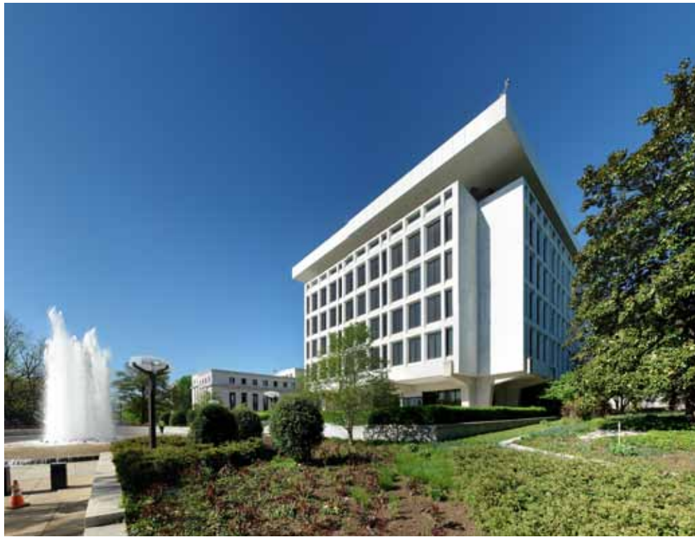
3 NORTH EAST CORNER VIEW
