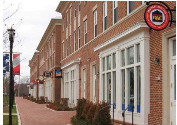
The Town Center along 12th Street serves as a model for mixed-use at the Post that can be expanded upon.
