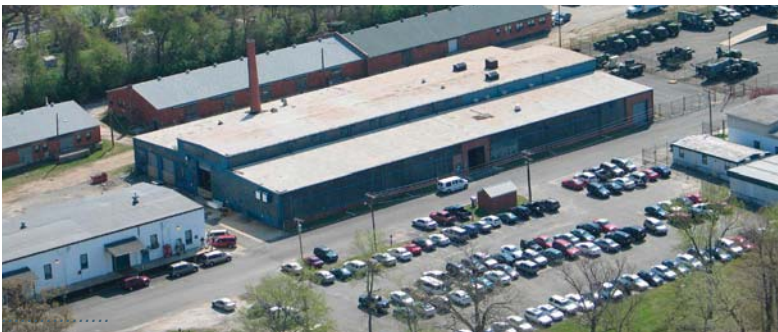
Industrial Area Neighborhood
