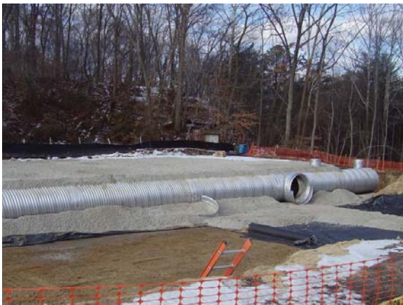
Installation of the underground detention system along Pohick Road.
