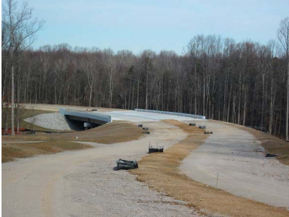
Construction of Mulligan Road, Fort Belvoir
