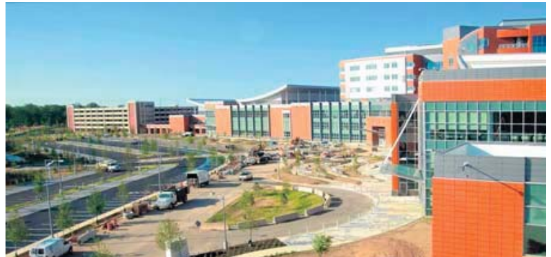
Hospital Under Construction
