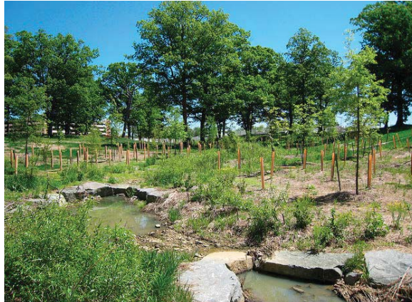
This stream was engineered to reduce water flow and allow runoff particulates to settle out in larger pools as part of the Fort Belvoir stream restoration efforts. (Photo by Gregory W. Fleming, Fort Belvoir DPW-ENRD)
