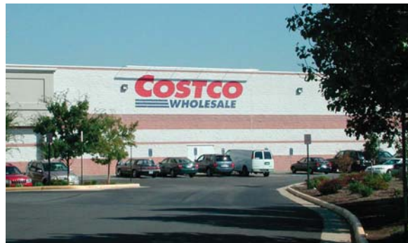
Industrial Area south of FBNA
