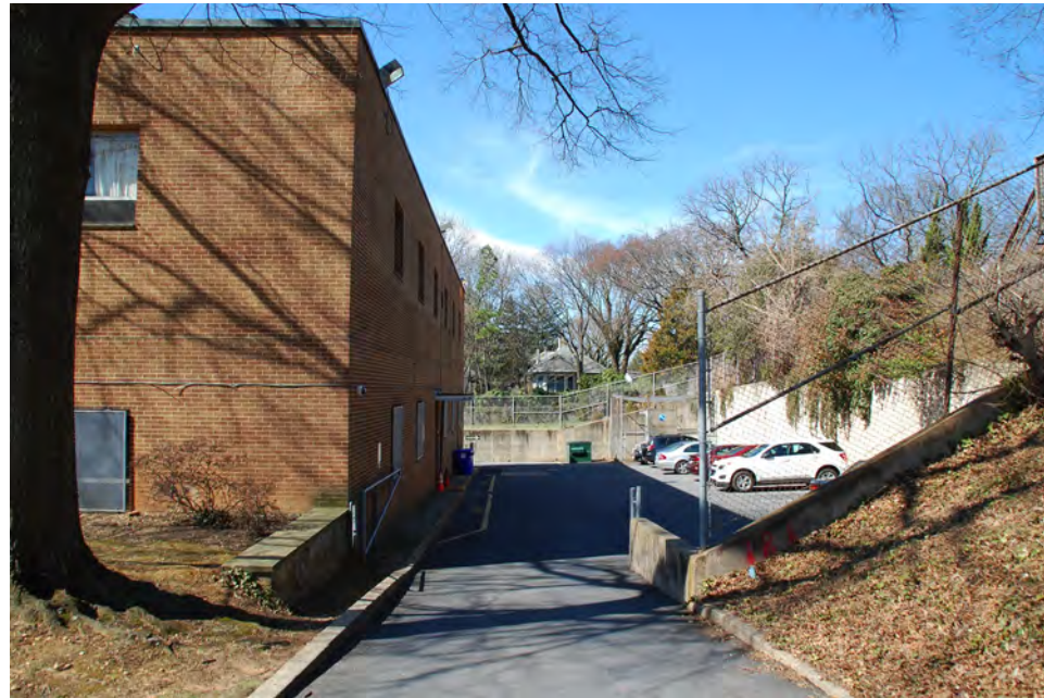
4 View of NE Corner and Parking
