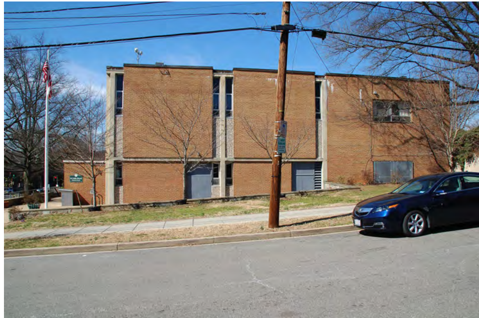
3 View of East Facade
