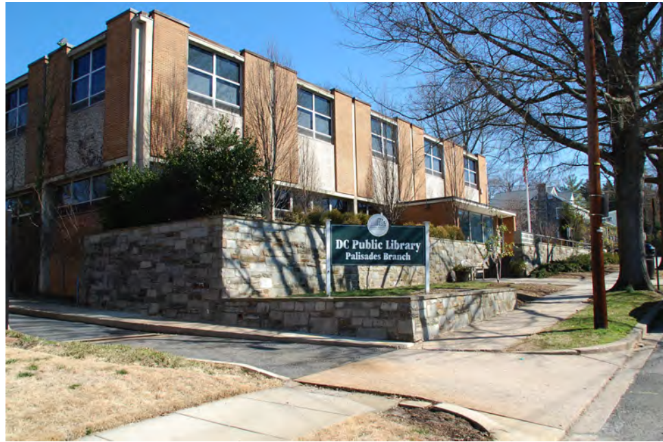
1 View of SW Corner
