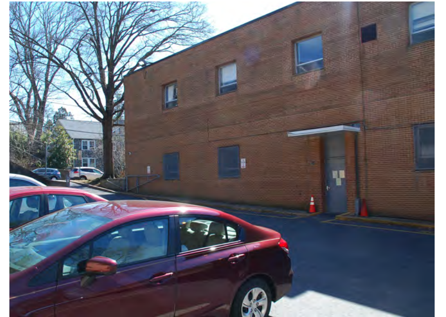
5 View of North Facade
