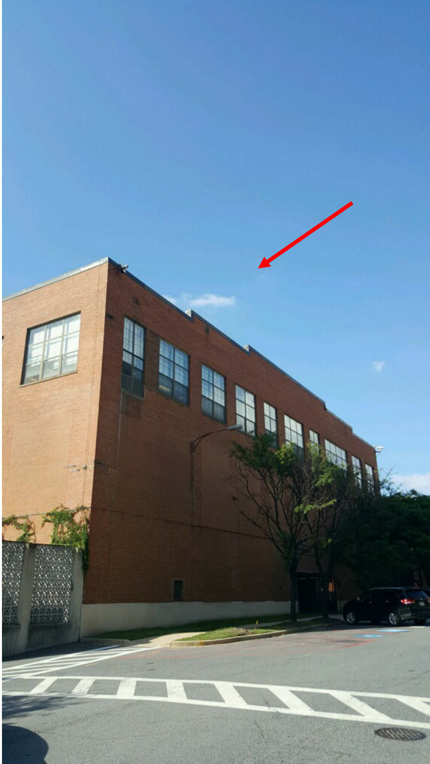
Bldg 196 from 10 th Street
