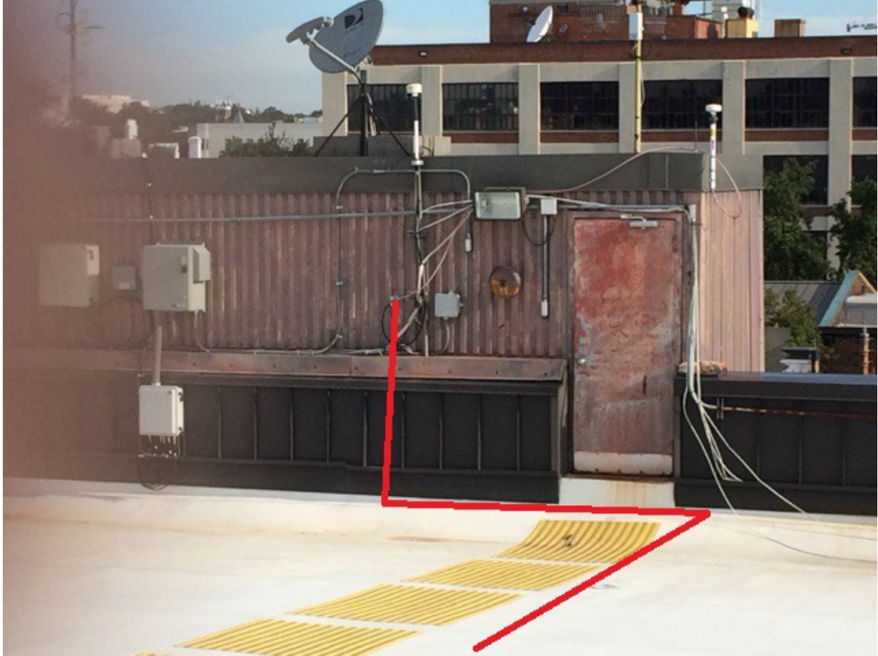
Looking east, red line indicates conduit route.
