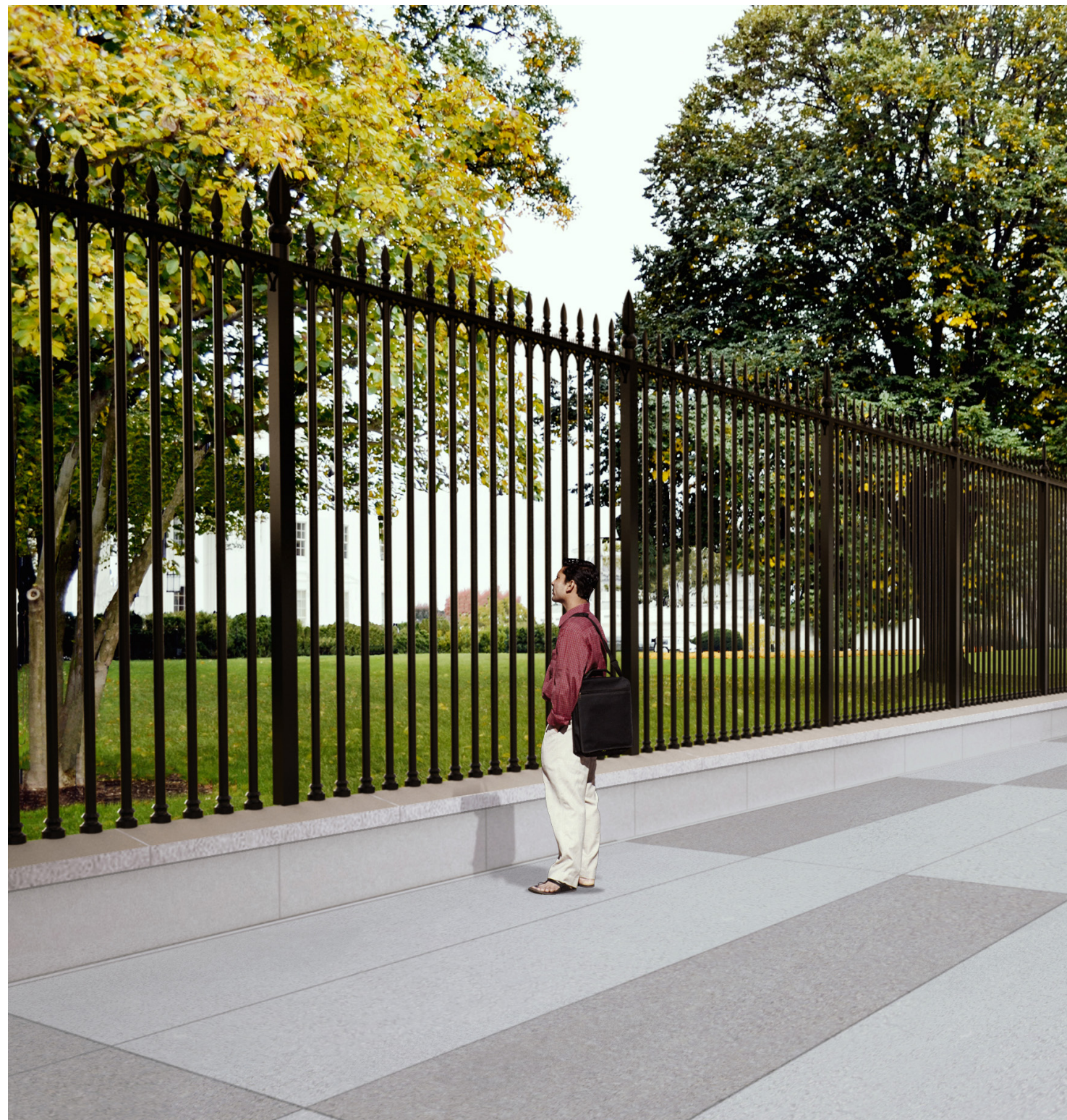
North side along Pennsylvania Avenue Concept A (2" pickets with 5 1/2" clear space)
