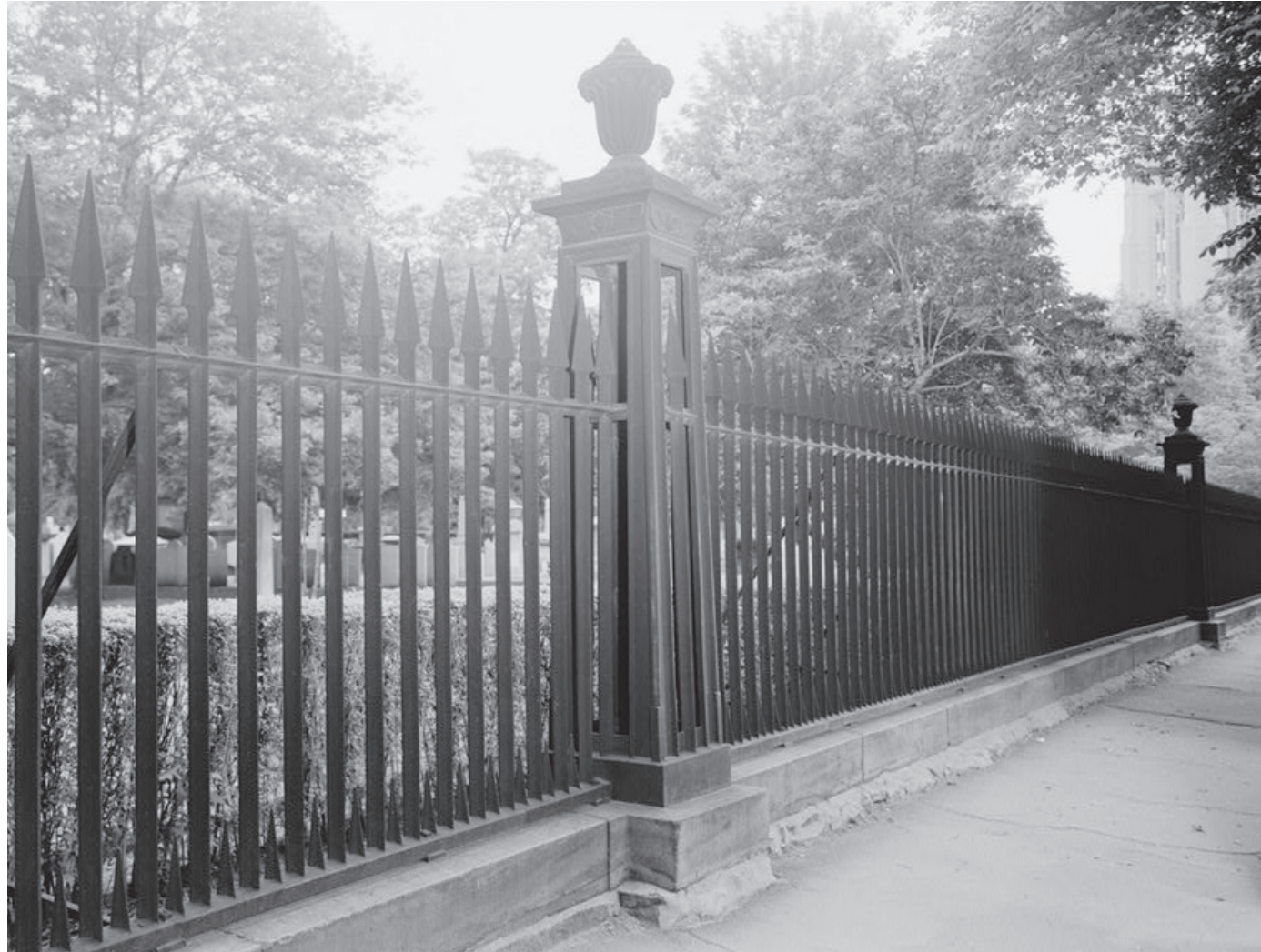
Grove Street Cemetery | New Haven, CT (7' fence, 1 1/2" square iron pickets, 4 1/2" clear space)
