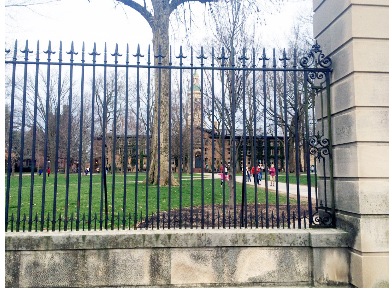
Nassau Hall | Princeton, NJ (36" base, 10' fence, 1" square iron pickets, 4" clear space)
