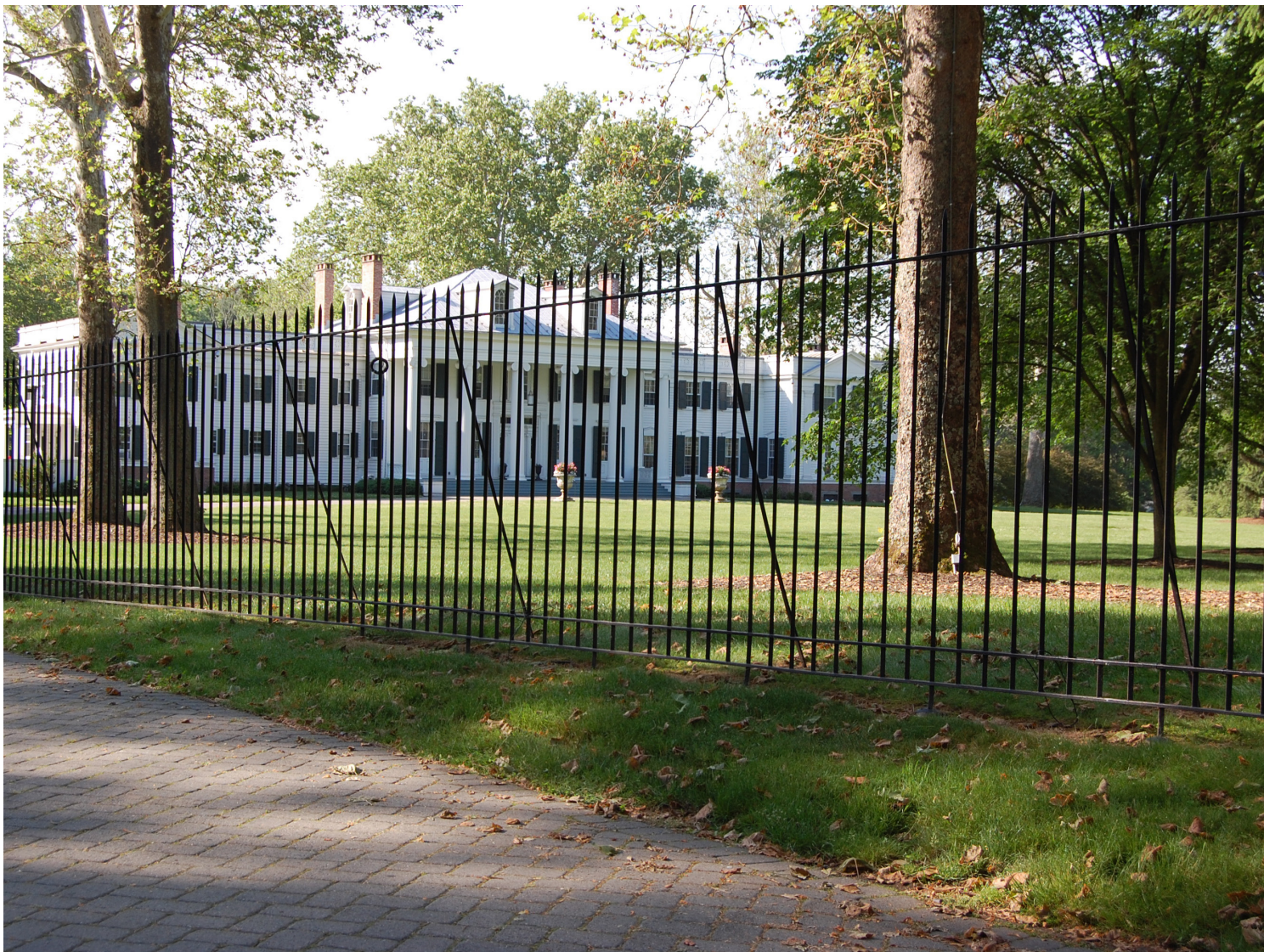
Drumthwacket | Princeton, NJ (7' high overall, 3/4" square iron pickets on diagonal, 5 1/2" clear space)
