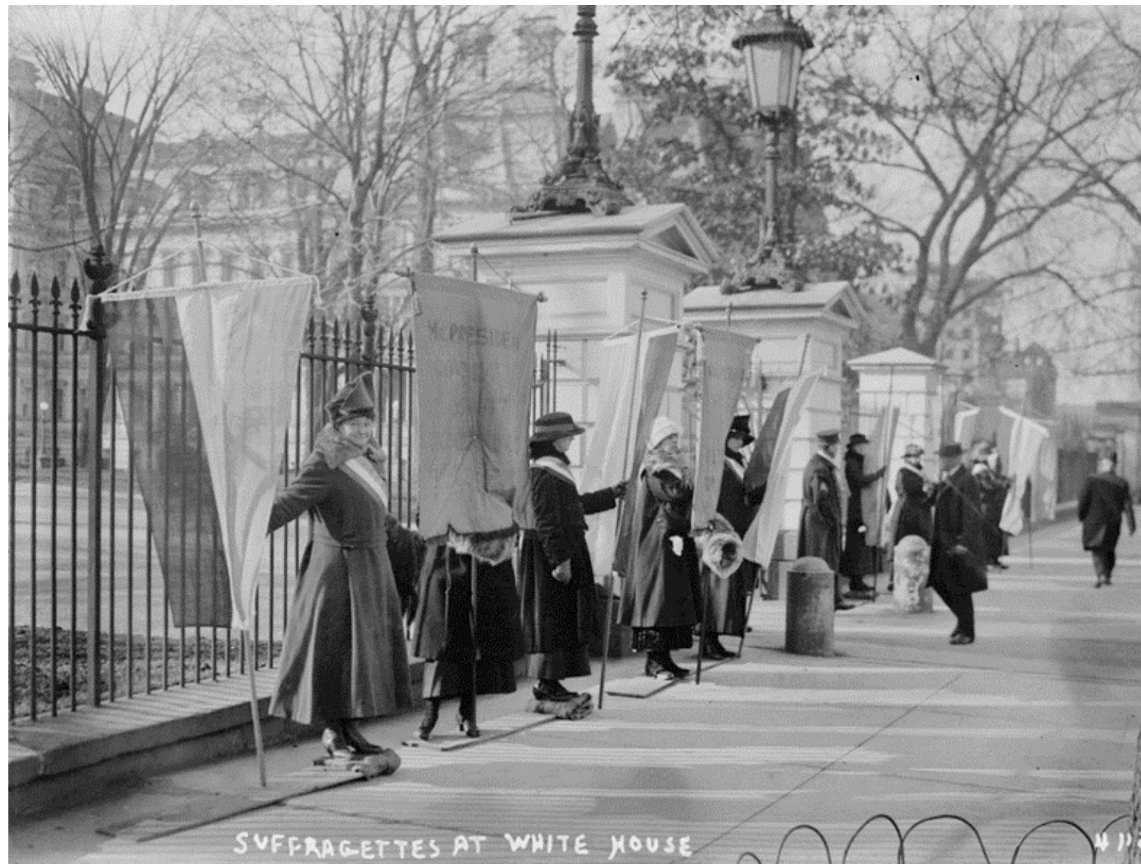
Photo ca. 1915 Fence attains current form between 1900 & 1920
