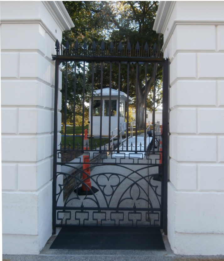
Pedestrian Gate Pennsylvania Ave
