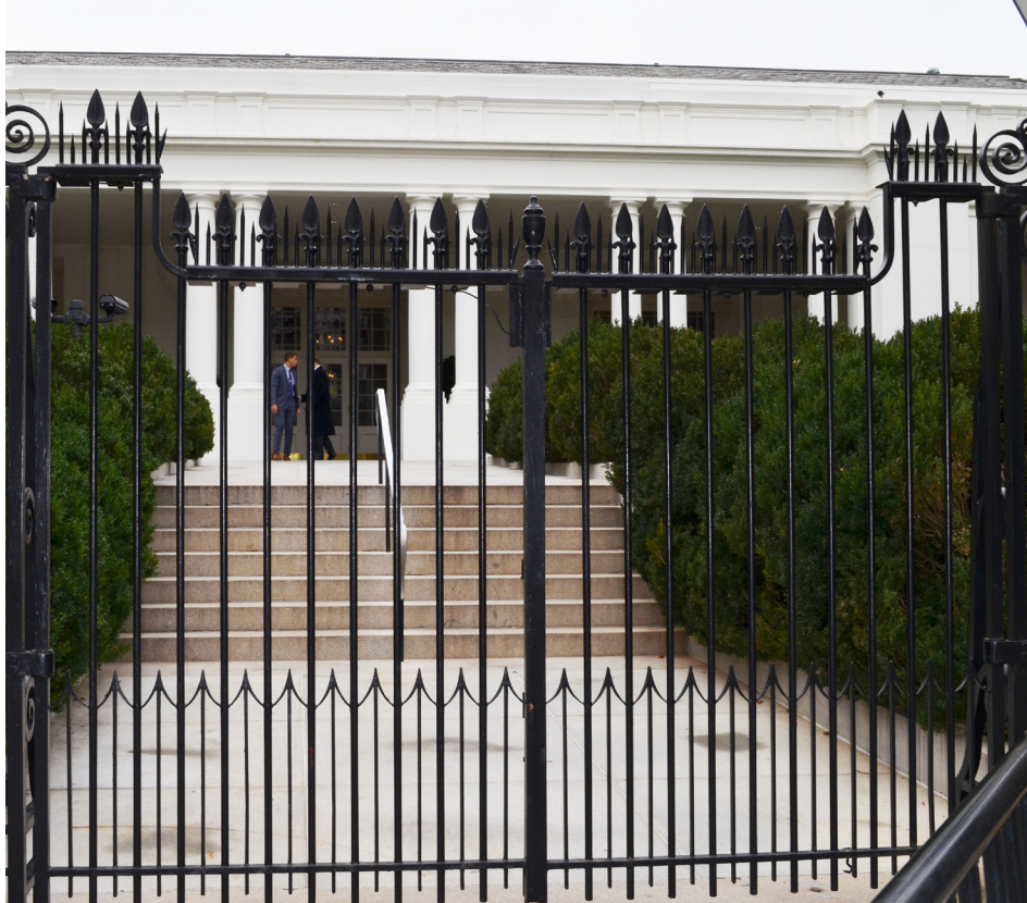
Visitor Entrance Gate East Executive
