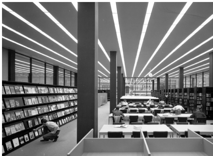
First floor west reading room, facing southeast, circa 1972. DCPL Archives.
