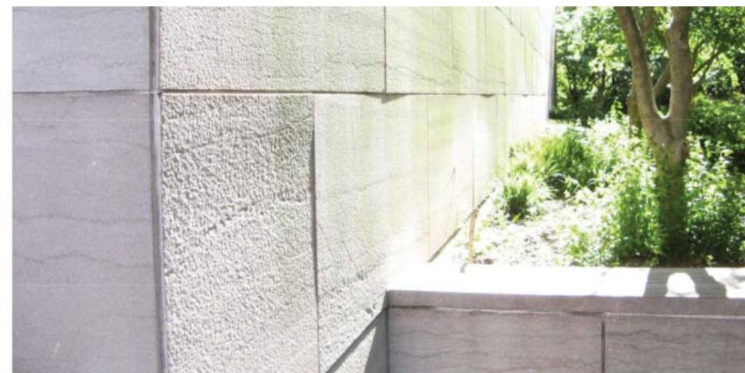
Warped Stone Panels on West Facade
