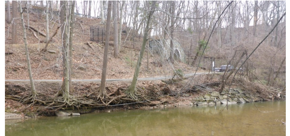
The northeast bank of Rock Creek in vicinity of the pedestrian bridge is eroding during heavy storms and undermining the existing trail.
