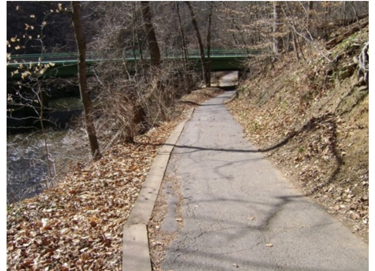
Existing Timber Edge Support
