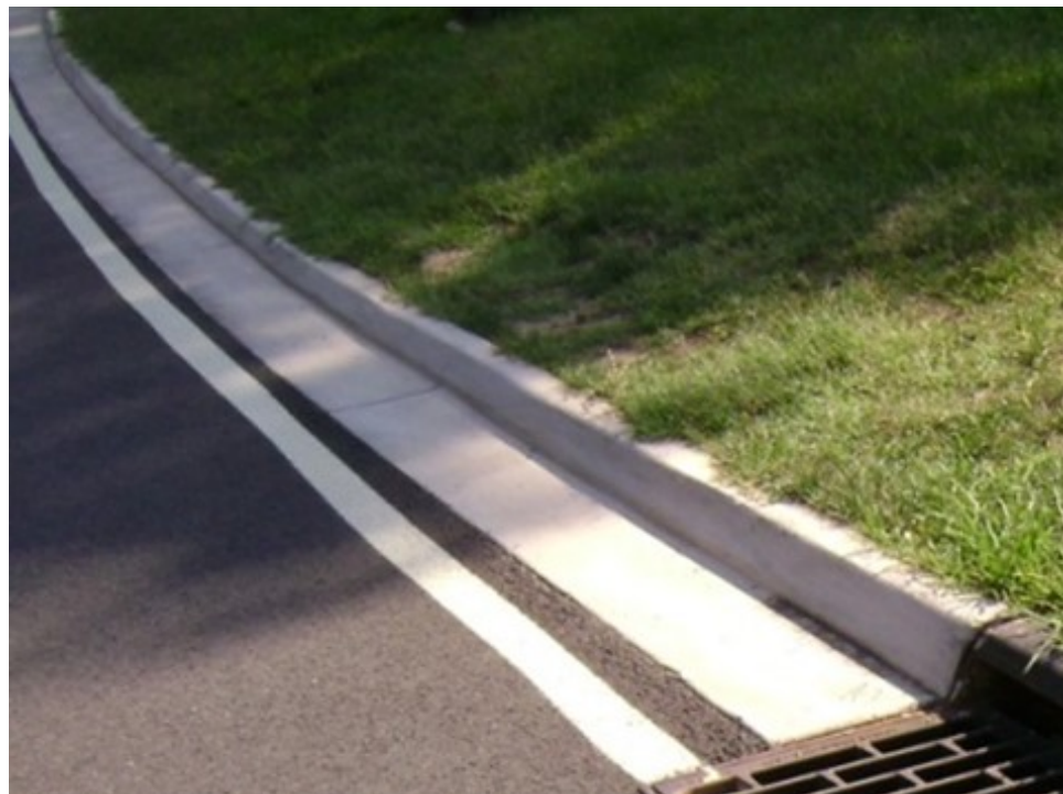
Existing Concrete Curb and Gutter
