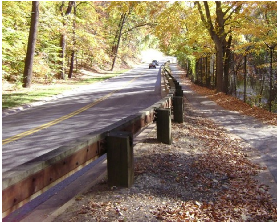
Existing Timber Steel Backed Timber Barrier
