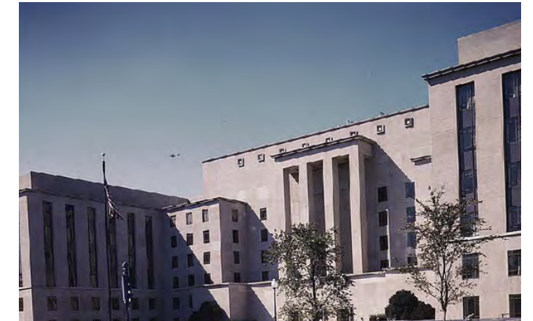
Figure 3-G. The east façade of the War Department Building, circa 1943. The original entrance, visible behind the tree in the center of the photograph, consisted of three doorways beneath the central portico. (Library of Congress, Prints and Photographs Division, LC-USW36-750, http://lcweb2.loc.gov )
