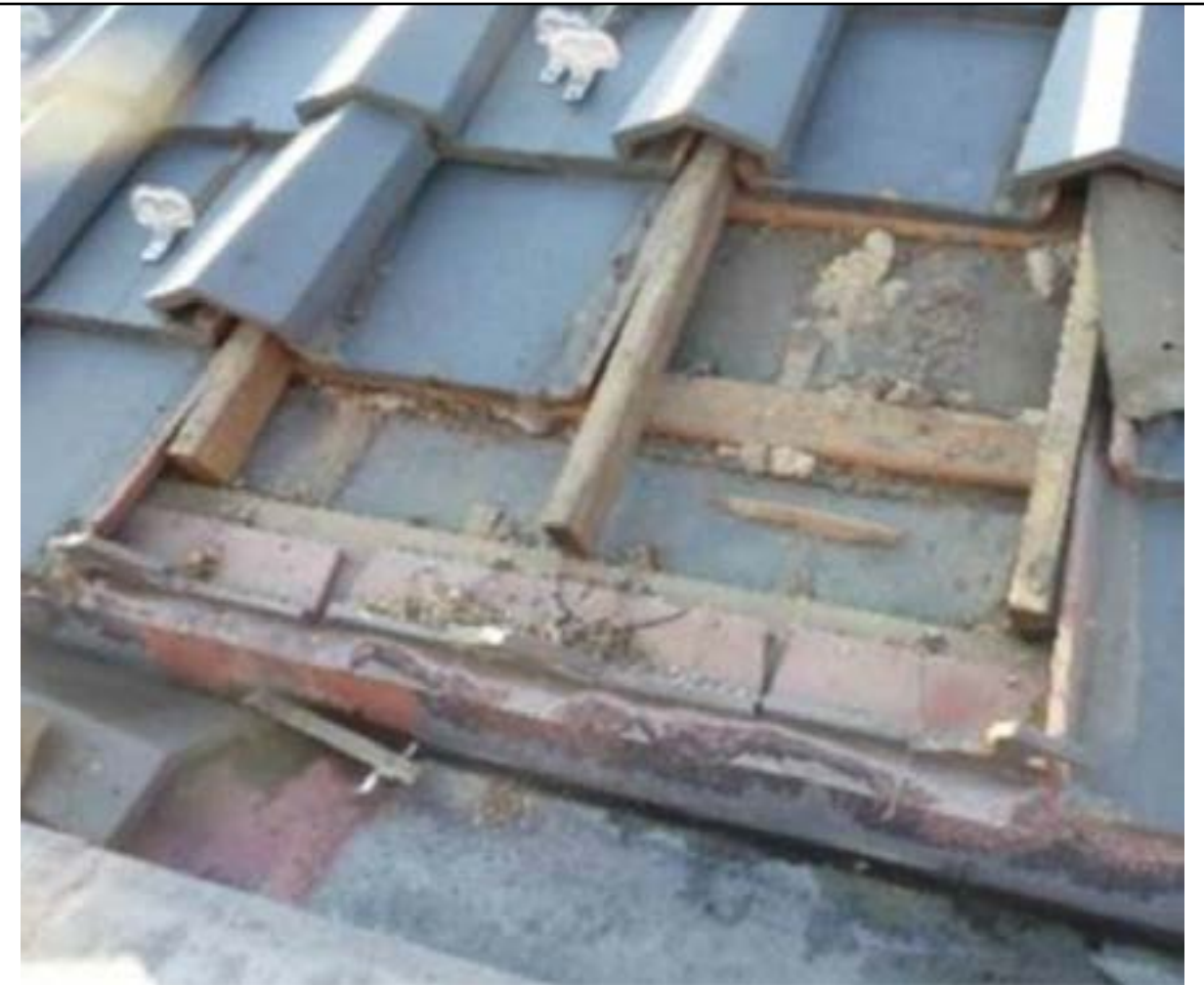
DETAIL VIEW OF ROOF ASSEMBLY
