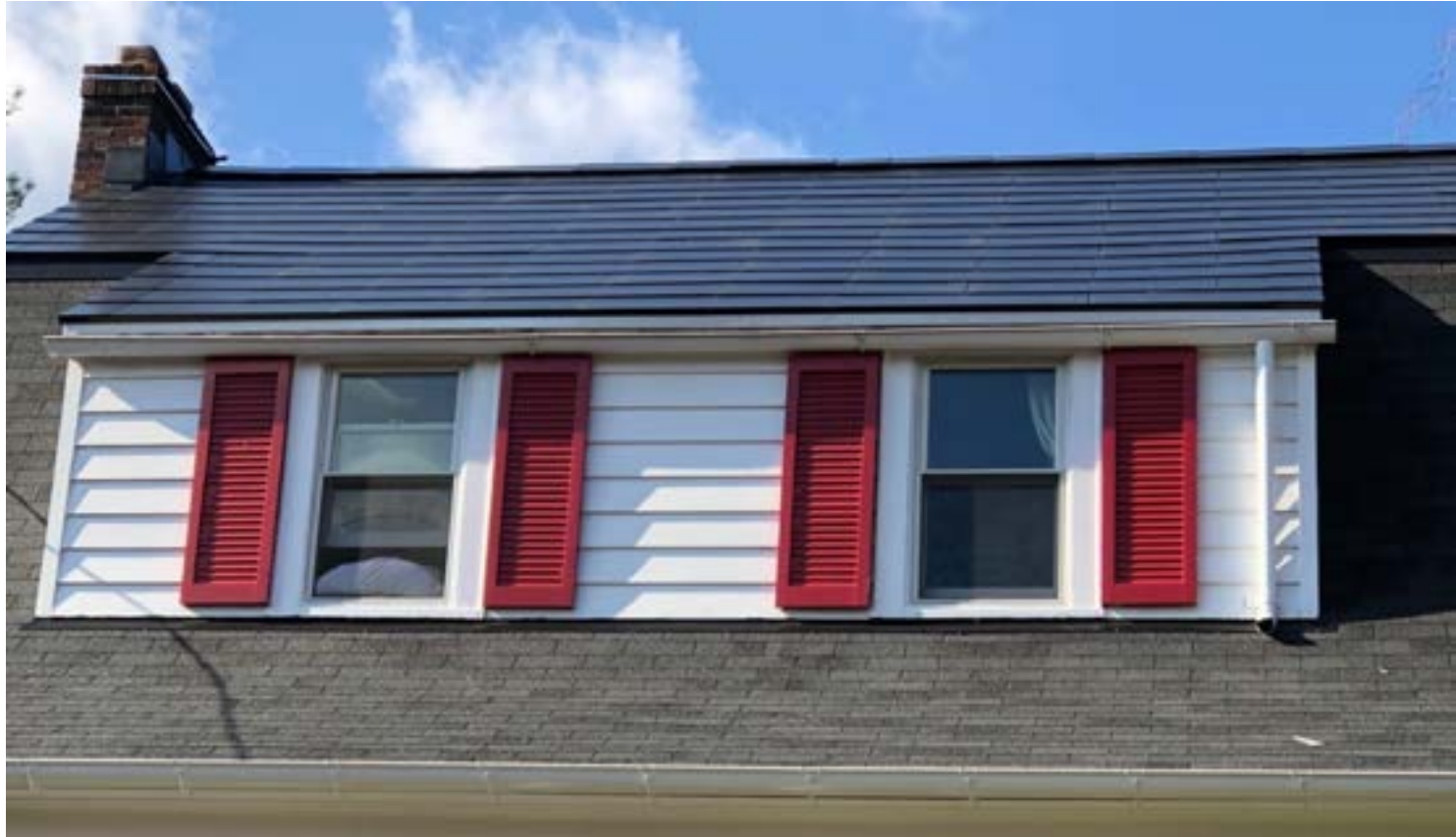
VIEW OF SOLAR TILE ROOF EDGE
