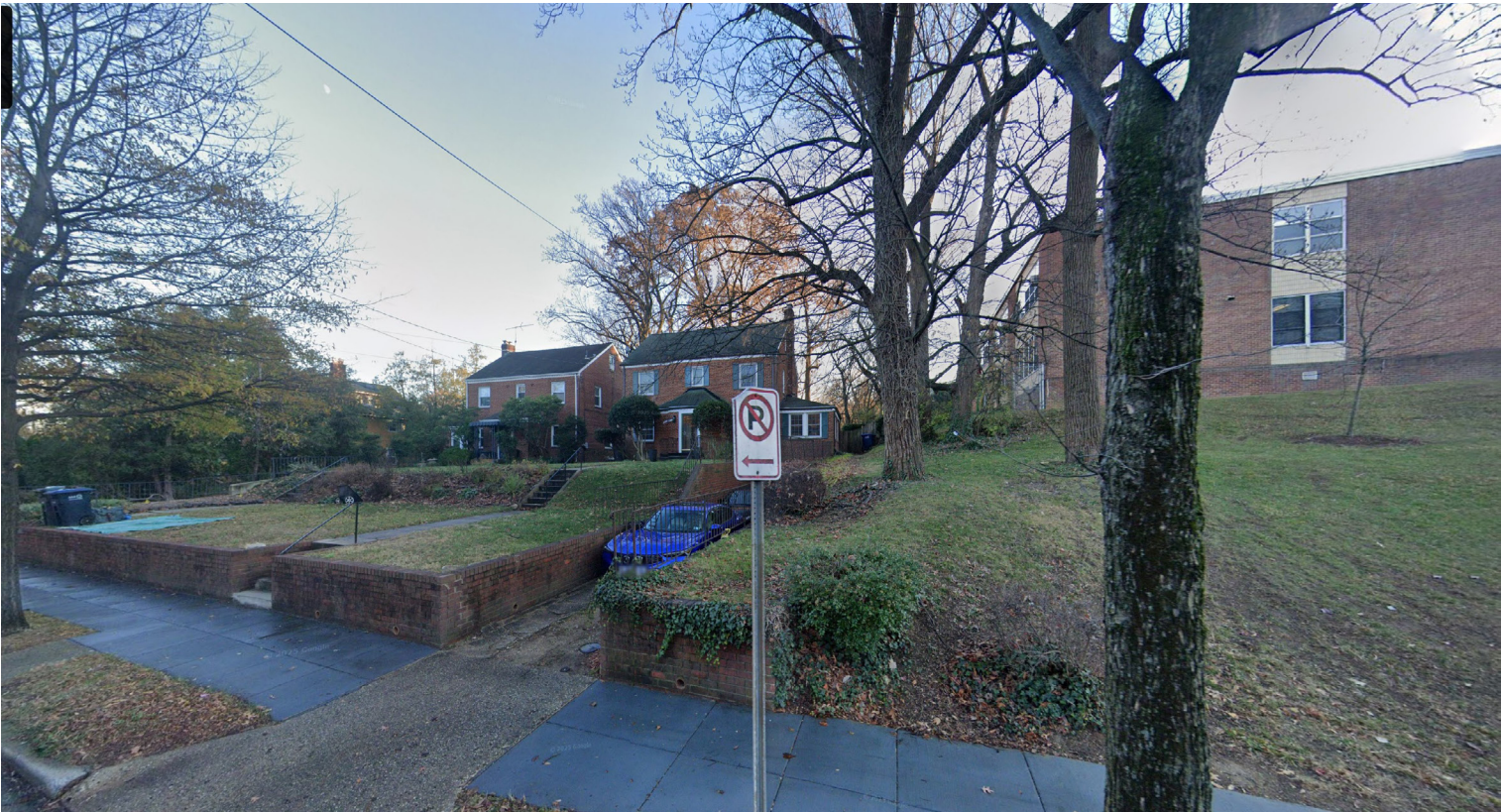
MICHIGAN AVE - ADJACENT BUILDINGS
