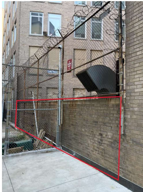
Figure 2 Existing Brick Wall in Alley
