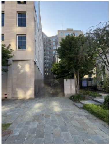
4 - STREET VIEW FROM 16TH ST SIDE WALK
