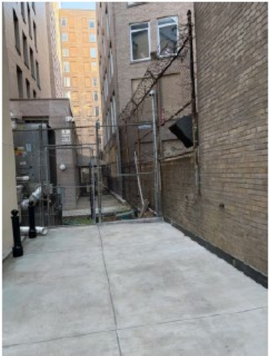
2 - EXISTING GATE INSIDE ALLEY
