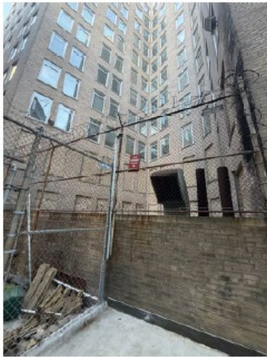
5 - VIEW INTO AIR SHAFT FROM ALLEYWAY LEVEL
