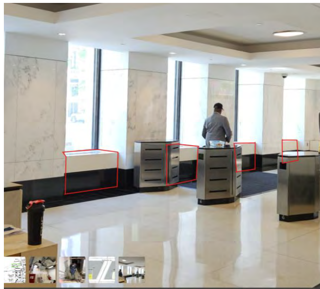
Figure 4 Fan Coil Unit Enclosures
