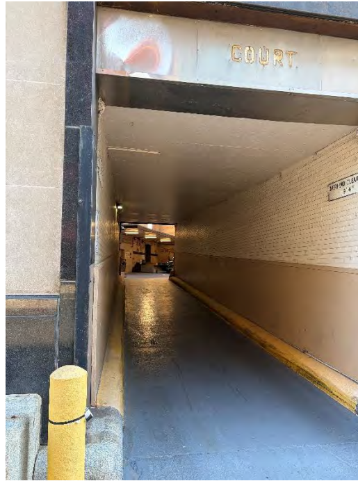
Figure 6 Under Building Tunnel to Loading Dock Area Taken from Sidewalk on H Street.
