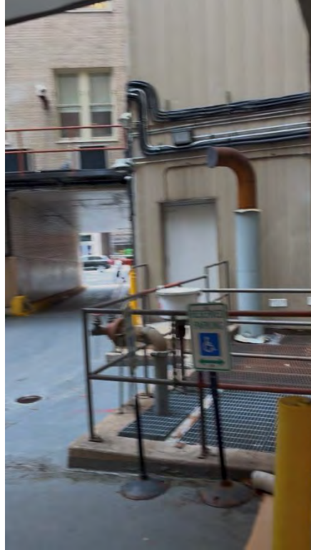
Figure 3 Light Well Next to Loading Dock Door and Access Tunnel Viewed from Loading Dock Area
