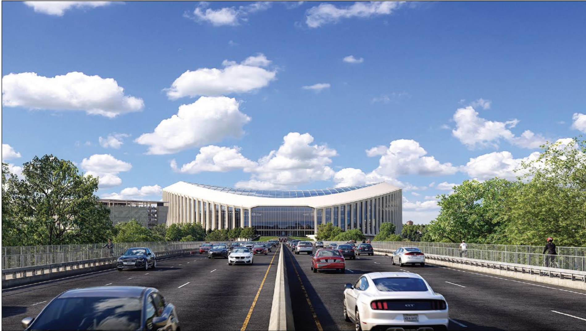
BRIDGE VIEW - EAST OF KINGMAN ISLAND
