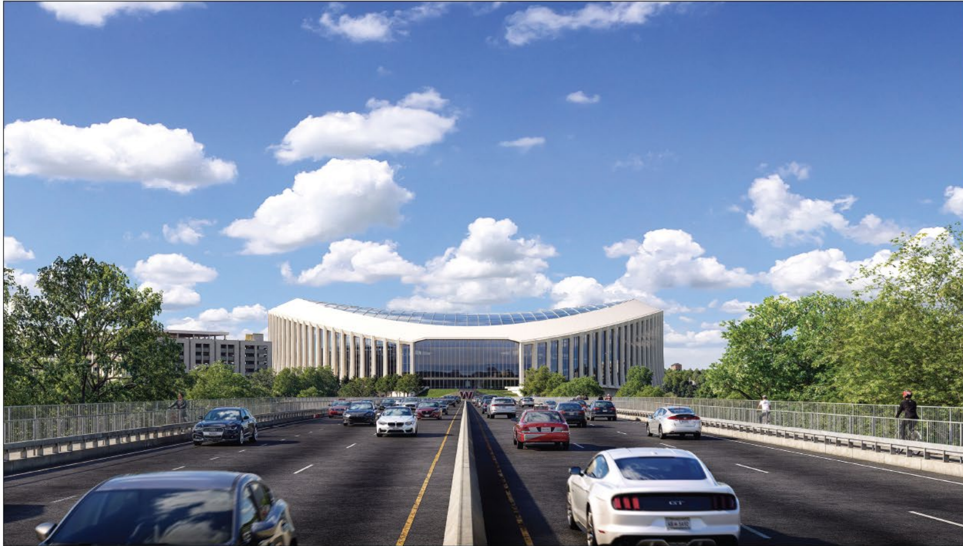
BRIDGE VIEW - EAST OF KINGMAN ISLAND
