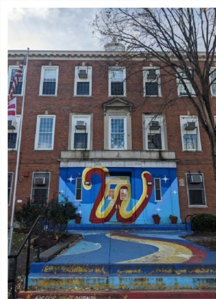
Paint TO BE REMOVED from Front Facade Cast Stone
