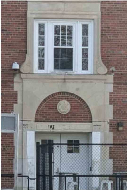
Historic Cast Stone on West Facade
