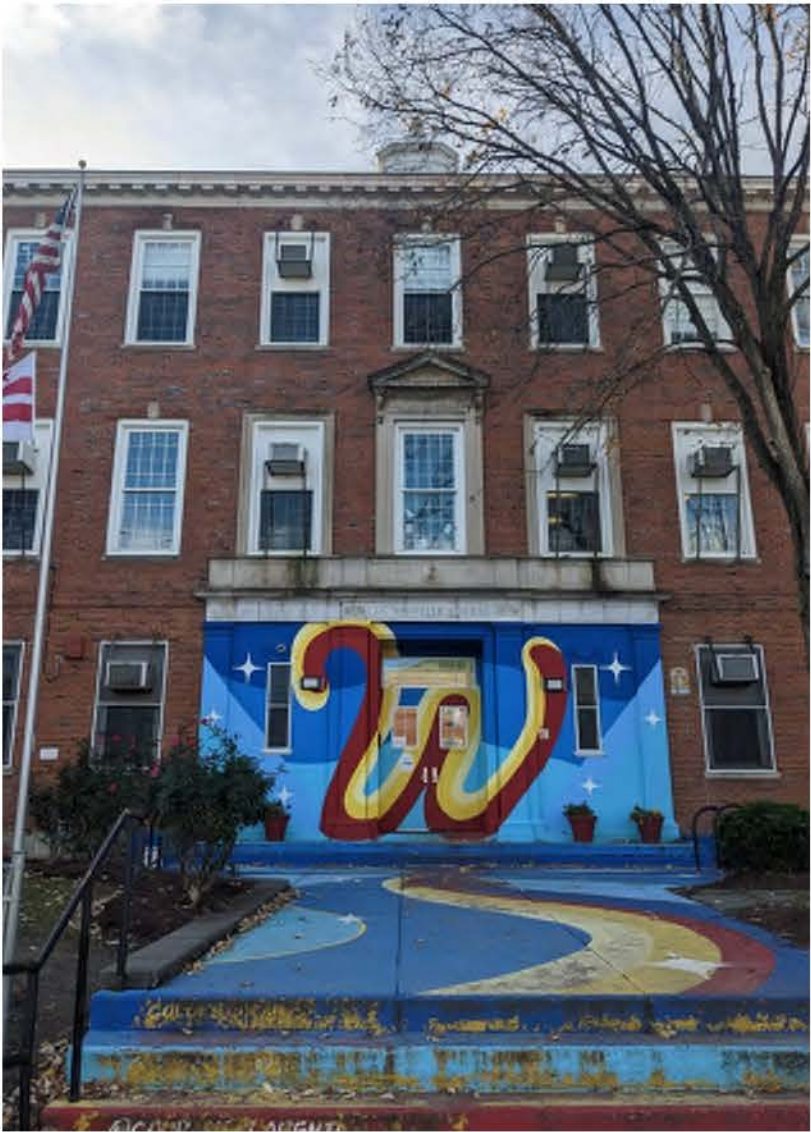
Paint TO BE REMOVED from Front Facade Cast Stone
