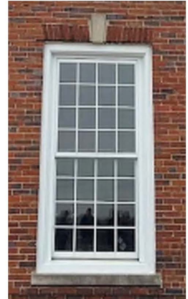
Current Windows w/ 16 over 16 lites. The proposed design will return to the 12 over 12 pattern from the historic photo.
