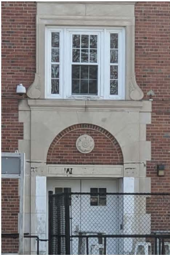
Historic Cast Stone on West Facade
