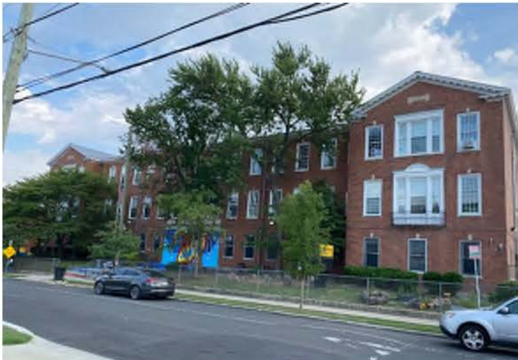
3. Main Entrance along Sheridan St.
