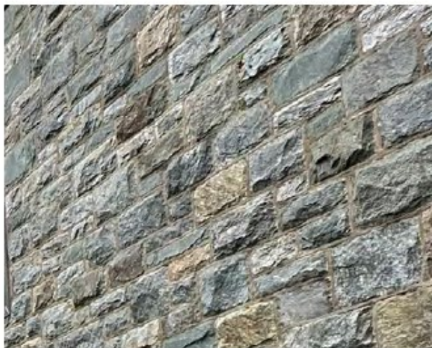
Figure 5.2.1.1: Proposed Facade Material Carderock, Ashlar Coursing
