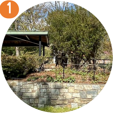
STONE RETAINING WALL
