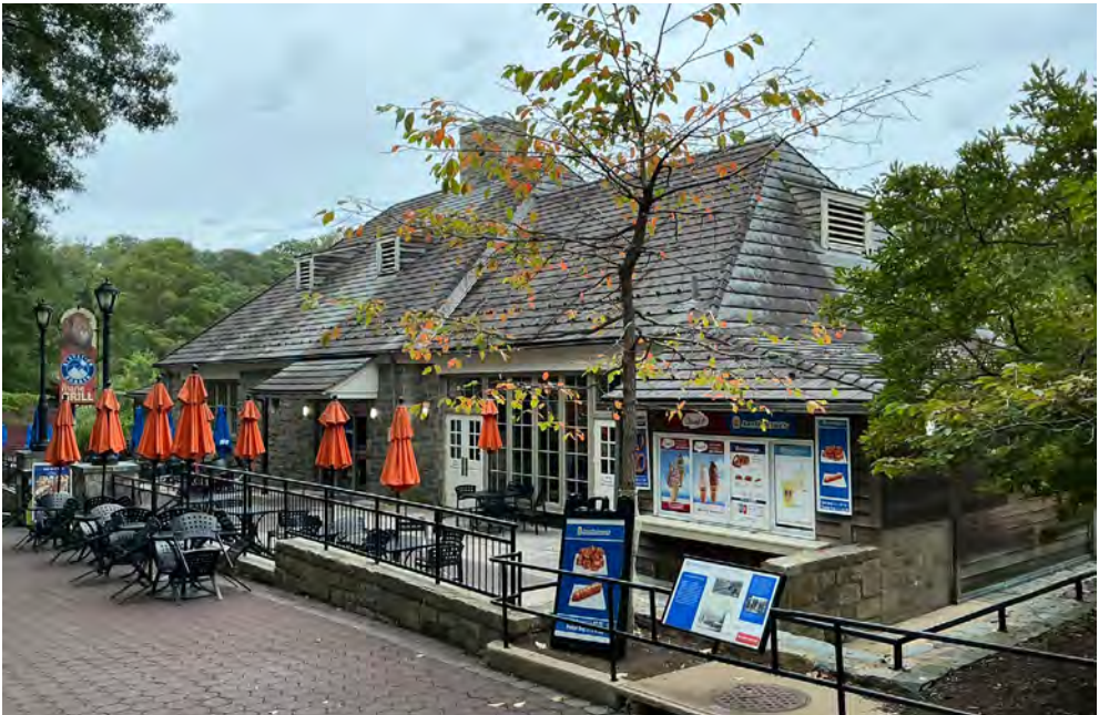
Figure 4.6.5.1: Existing Use of Stone and Roof Features
