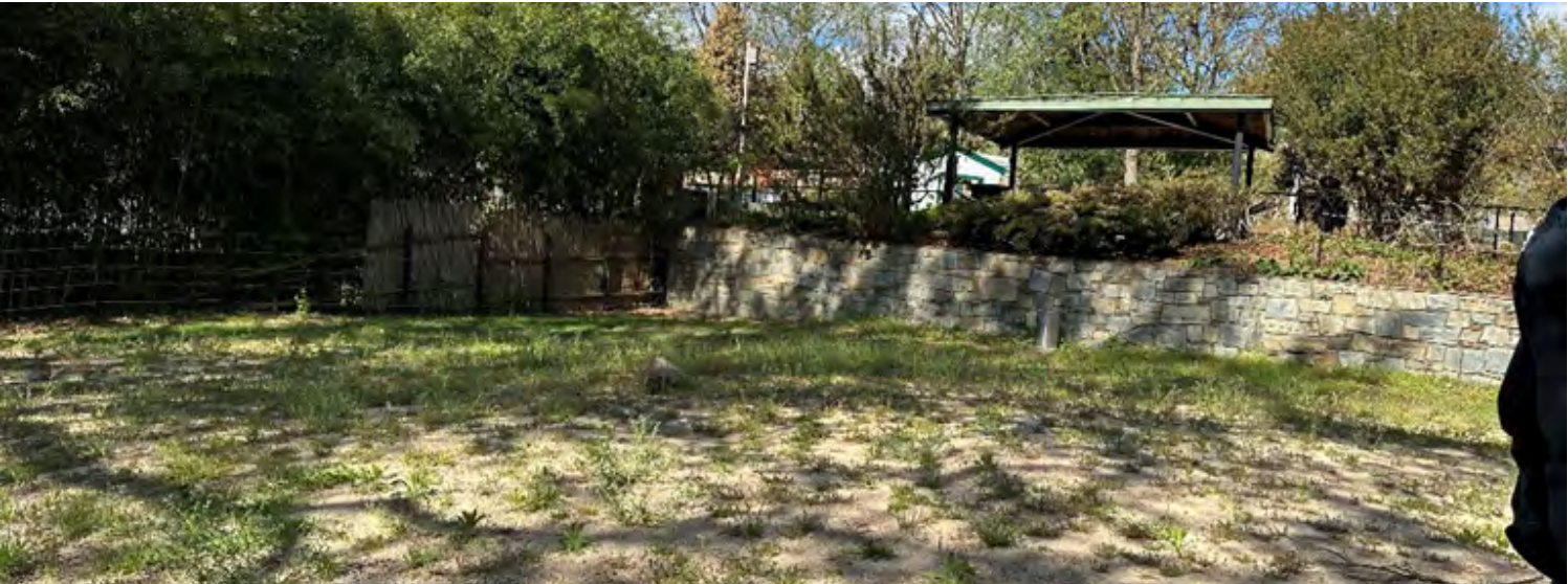
Figure 4.5.2.2: View from within Bison Habitat exhibit looking north to Zoo in Your Backyard exhibit, showing stone retaining wall, metal-roofed pavilion, deactivated electrical fence, tall bamboo, and typical sandy ground surface with sparse grass.
