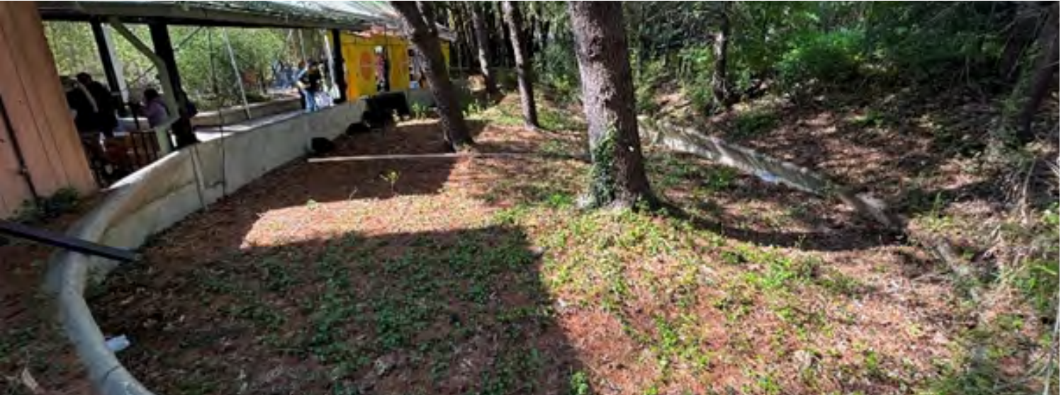
Figure 4.5.2.3: View from back of the Bison Care building looking south. The concrete retaining wall of the former prairie dog exhibit is filled with weeds and white pine trees. A metal-roofed pavilion covers a temporary panda-related vendor in the left background.
