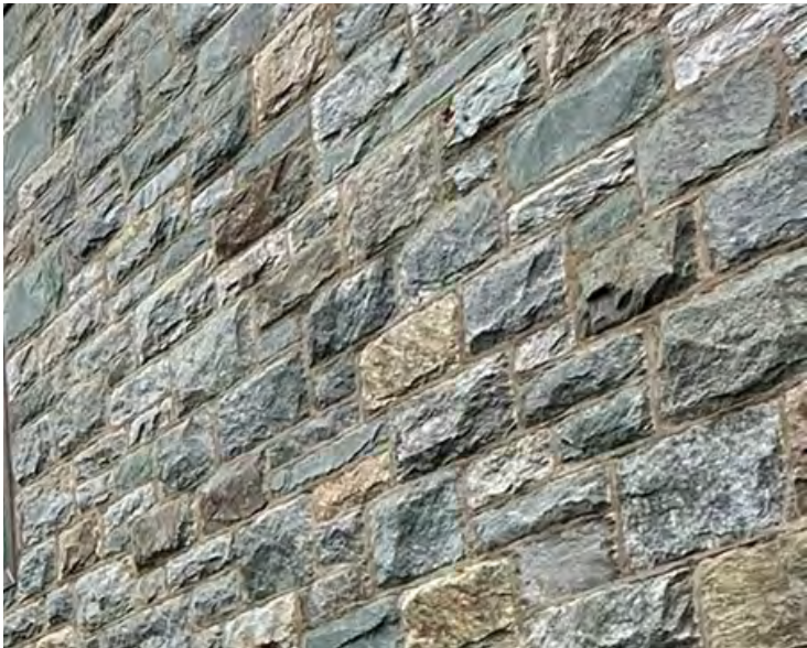
Figure 5.2.1.1: Proposed Facade Material Carderock, Ashlar Coursing
