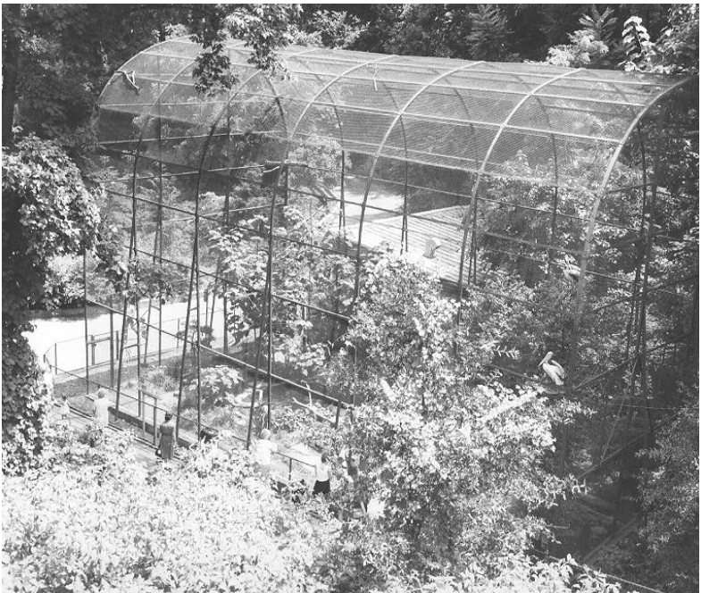
Figure 3.2.1.2: Bird Enclosure, c. 1912 Note: Mesh screen with tall, pointed-arch superstructure to accommodate animals' natural habitat and behavior (demolished)
