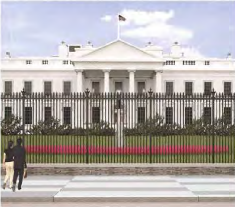
White House Fence
