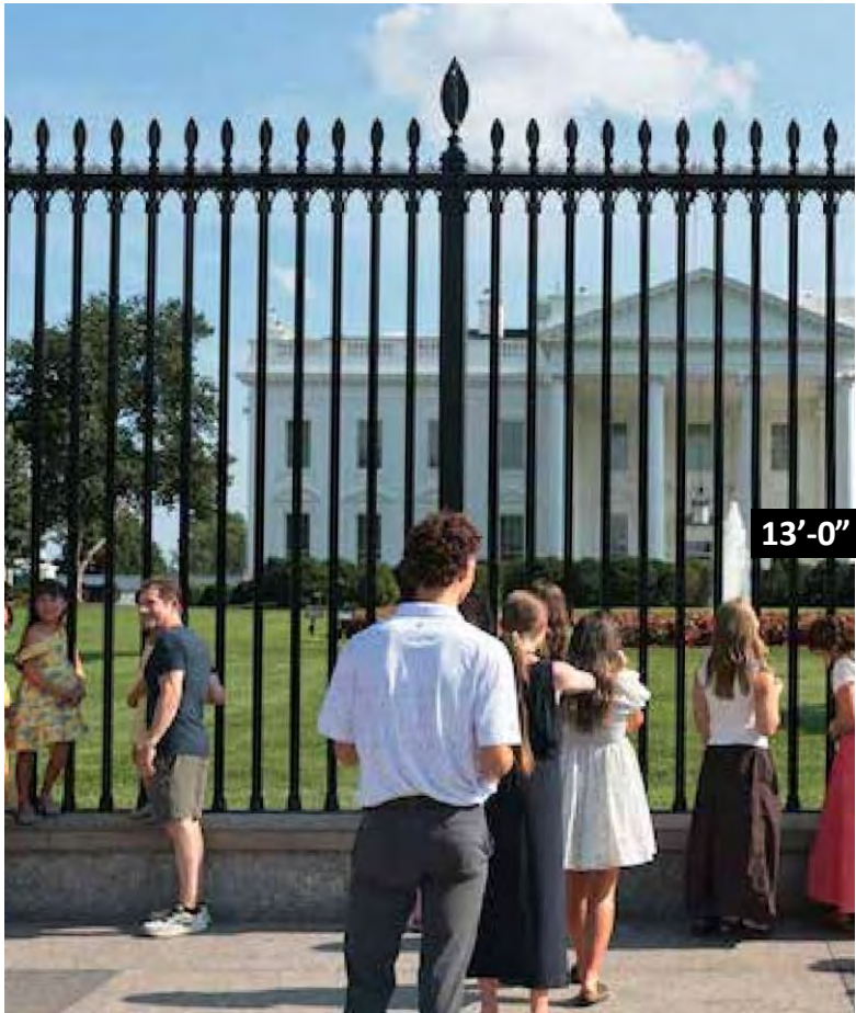
WHITE HOUSE FENCE
