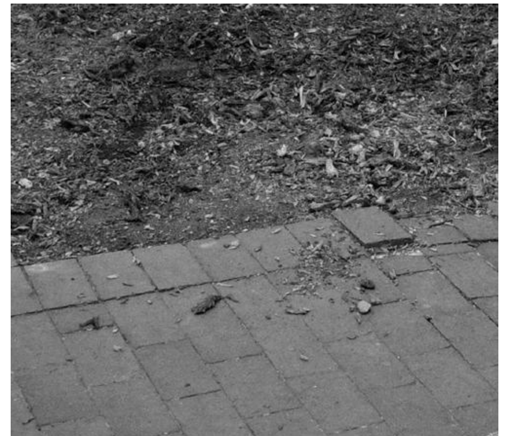
Site Visit Photos, 2026
