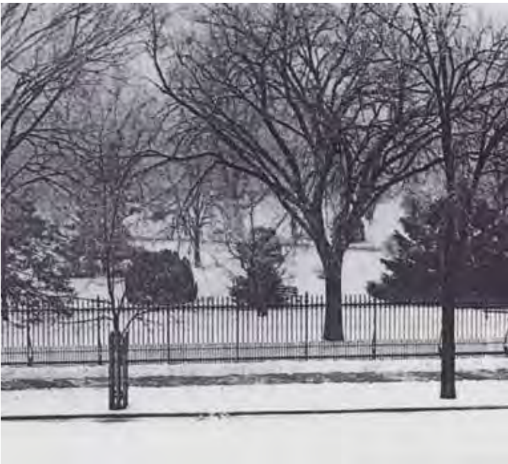
HISTORIC LAFAYETTE PARK FENCE
