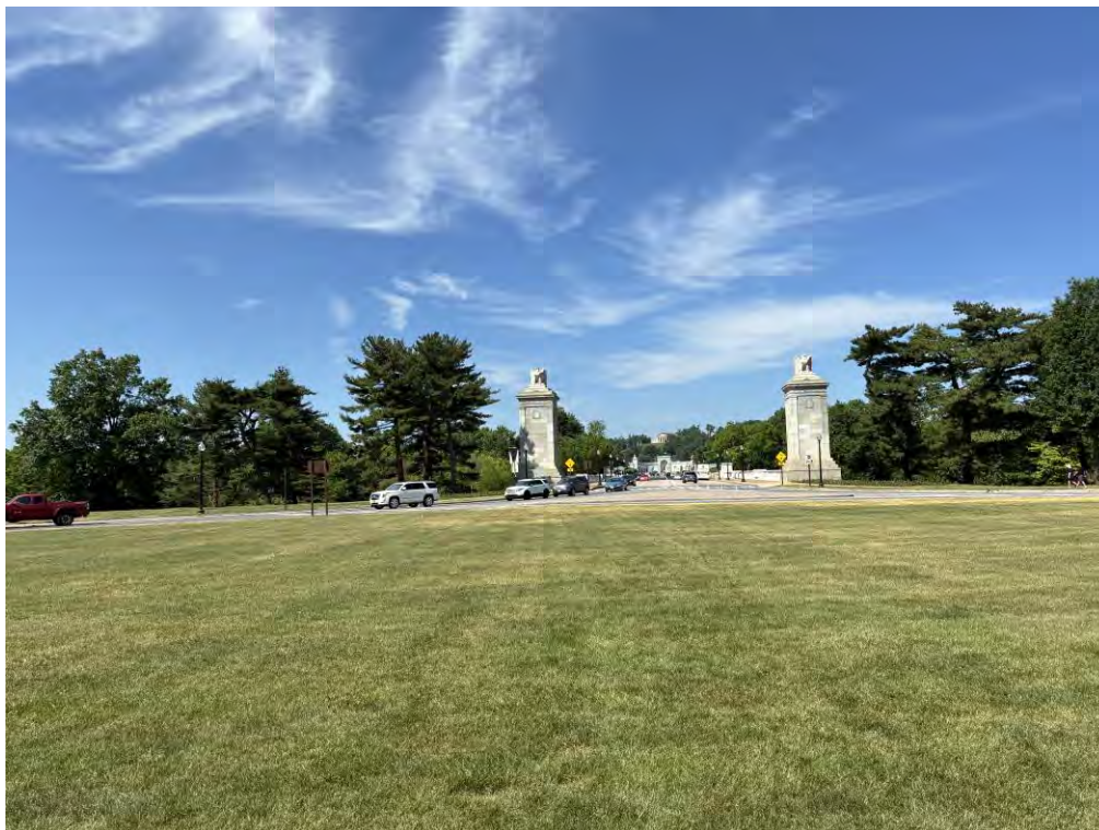
Photograph 5: Site Overview. Facing Southwest. BT 04/19/2026
