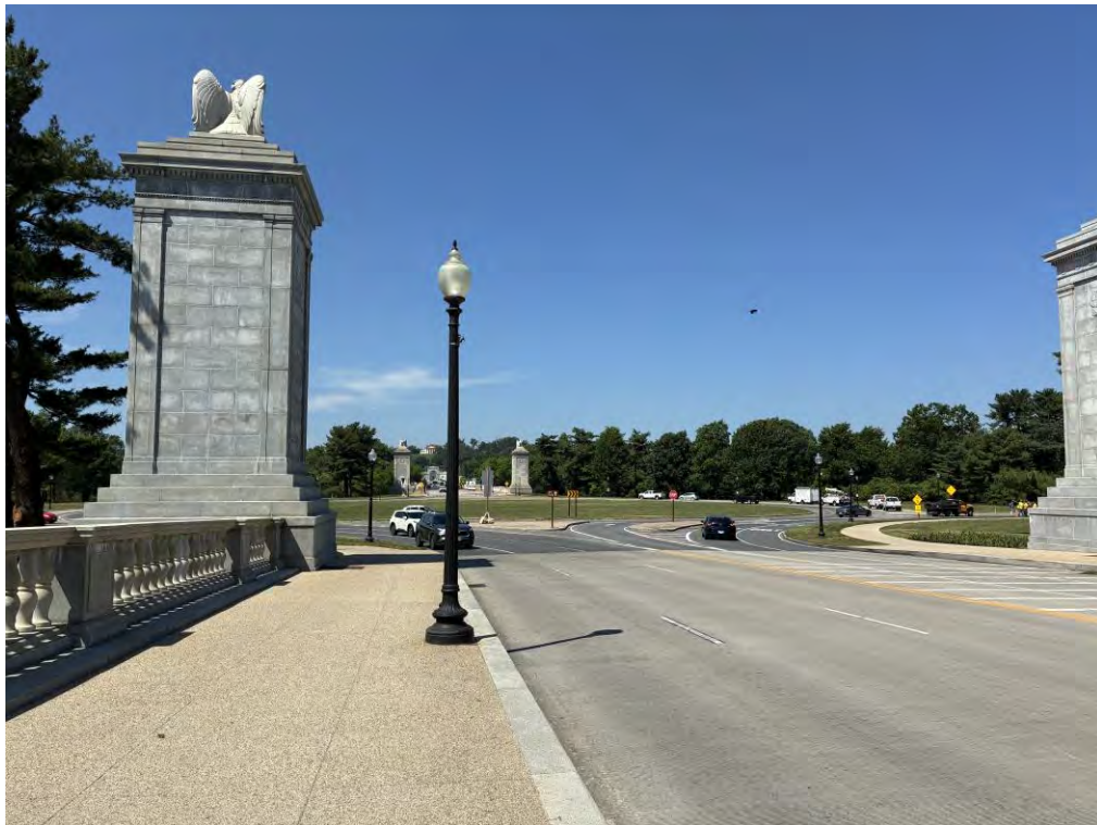
Photograph 18: Site Overview. Facing Southwest. BT 04/19/2026
