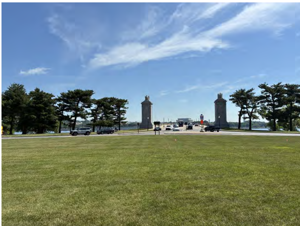
Photograph 2: Site Overview. Facing Northeast. BT 04/19/2026
