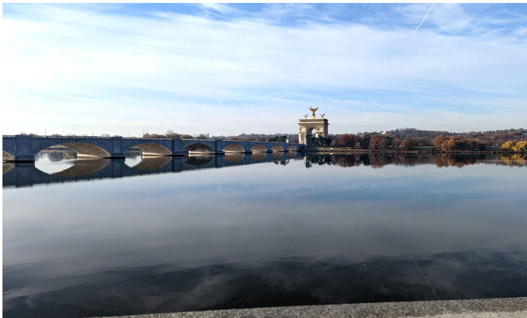
Image 13. View from the Parkway Dr. NW toward Arlington Memorial Bridge and Memorial Circle with the proposed Triumphal Arch. ©Harrison Design
