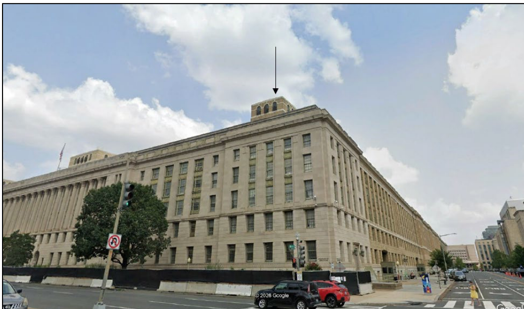
Figure 1: Southwest Corner Sector Antenna
