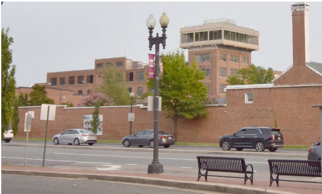
Figure 1: View of proposed Building 157 rehabilitation from M Street, SE.
