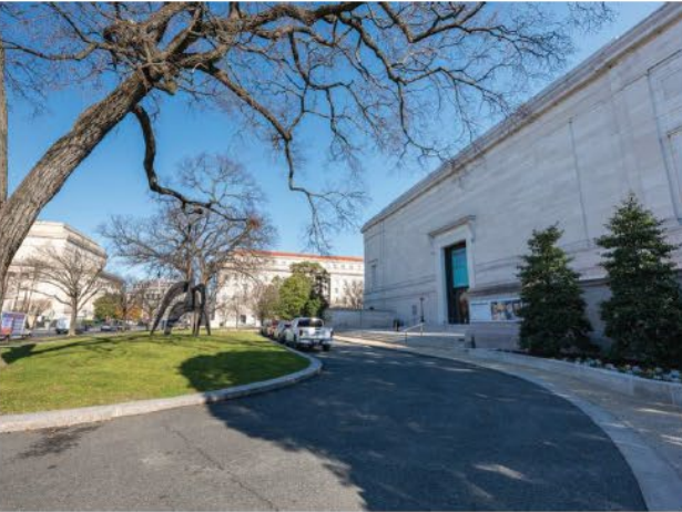
Figure 1-9. View of Seventh Street drive and center lawn panel.
