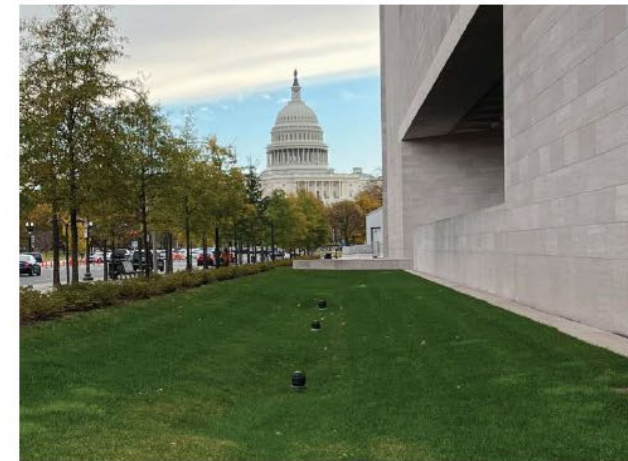
Figure 1-49. Image of existing bioretention at the National Gallery of Art East Building.
