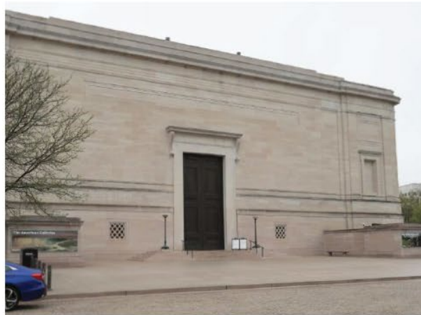
Figure 1-42. Marble landing and stairs and granite landing at the Fourth Street Entrance of the West Building.
