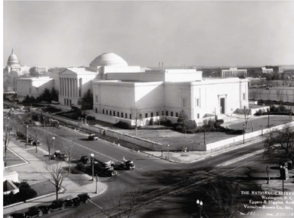
Figure 1-25. Construction progress on the West Building, November 1940. (National Gallery of Art, Washington, DC, Gallery Archives, RG26A, National Gallery of Art Architecture Images - West Building Original Construction, Photograph by Commercial Photo Co., 26A23_2289_001)
