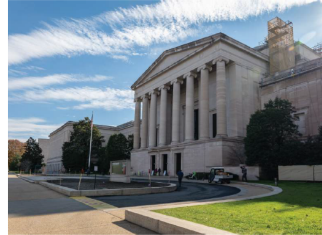
Figure 1-37. Ground-level view of the U-shaped vehicular and pedestrian routes to the Sixth Street Entrance.
