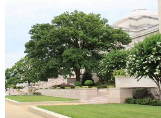
Figure 1-33. View looking west of the assemblage of lawn panels, stairs, site walls, and the courtyards and grand staircase beyond.
