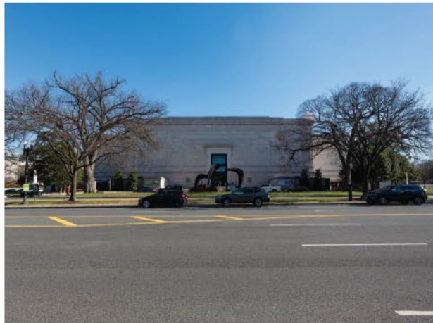
Figure 1-18. View of the Seventh Street Entrance from the entrance of the Sculpture Garden.
