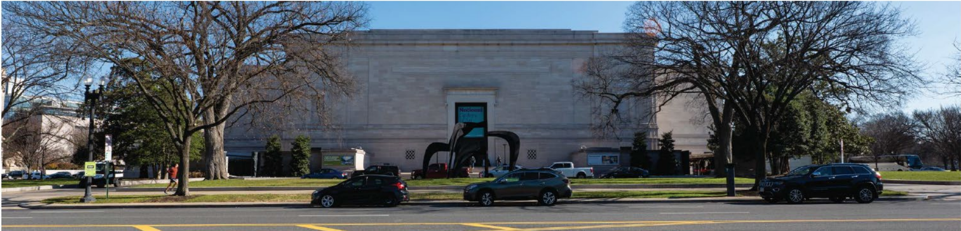
Figure 1-7. View of Seventh Street Entrance from Sculpture Garden Entrance.
