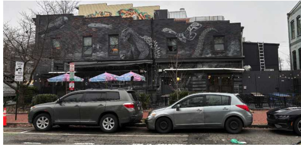
2 Q Street (East of Site)
