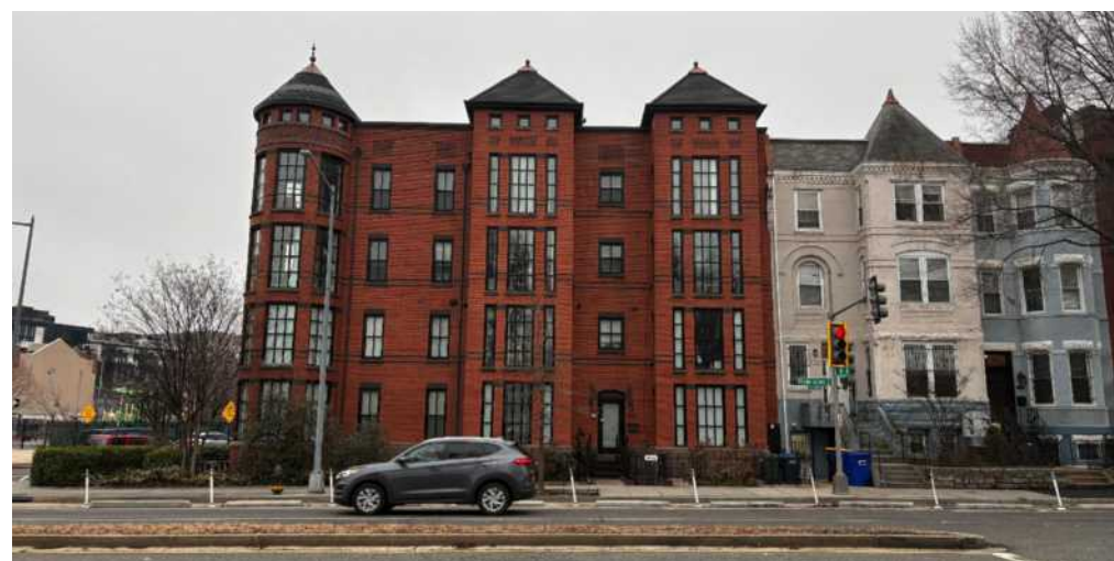
5 Residential Southern Side of Rhode Island
