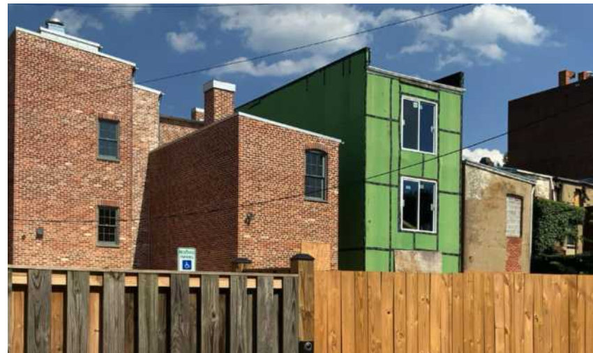
4 Rear of Adjacent Row Houses
