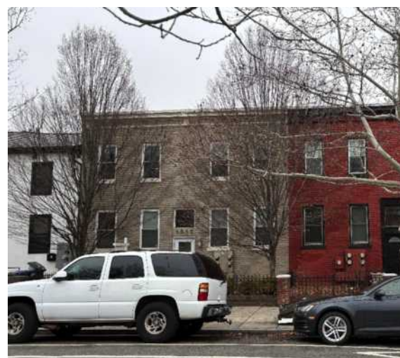
7 10th Street (Site Looking West)
