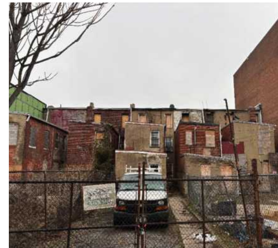
5 Rear of Adjacent Row Houses
