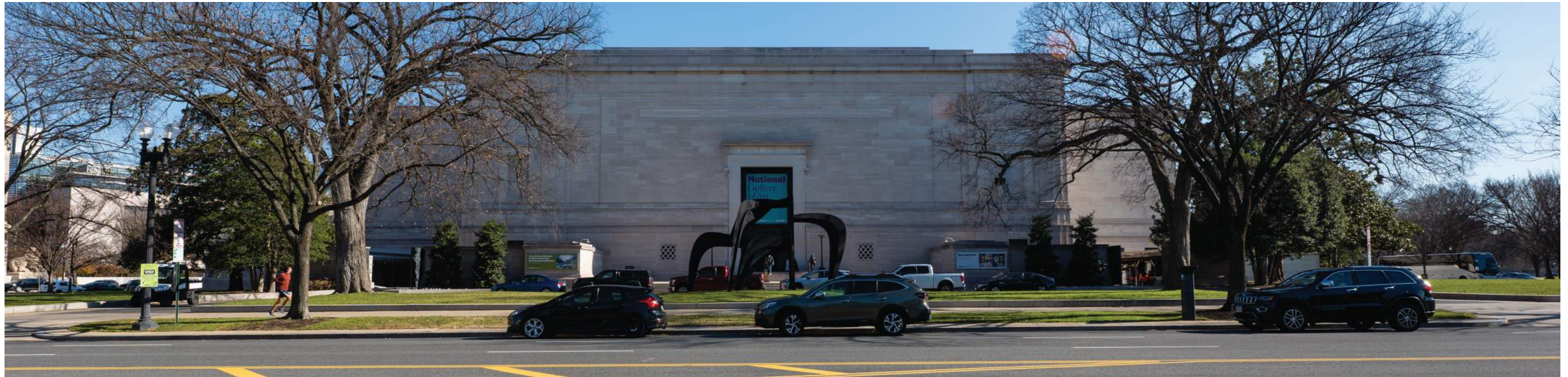
Figure 1-7. View of Seventh Street Entrance from Sculpture Garden Entrance.
