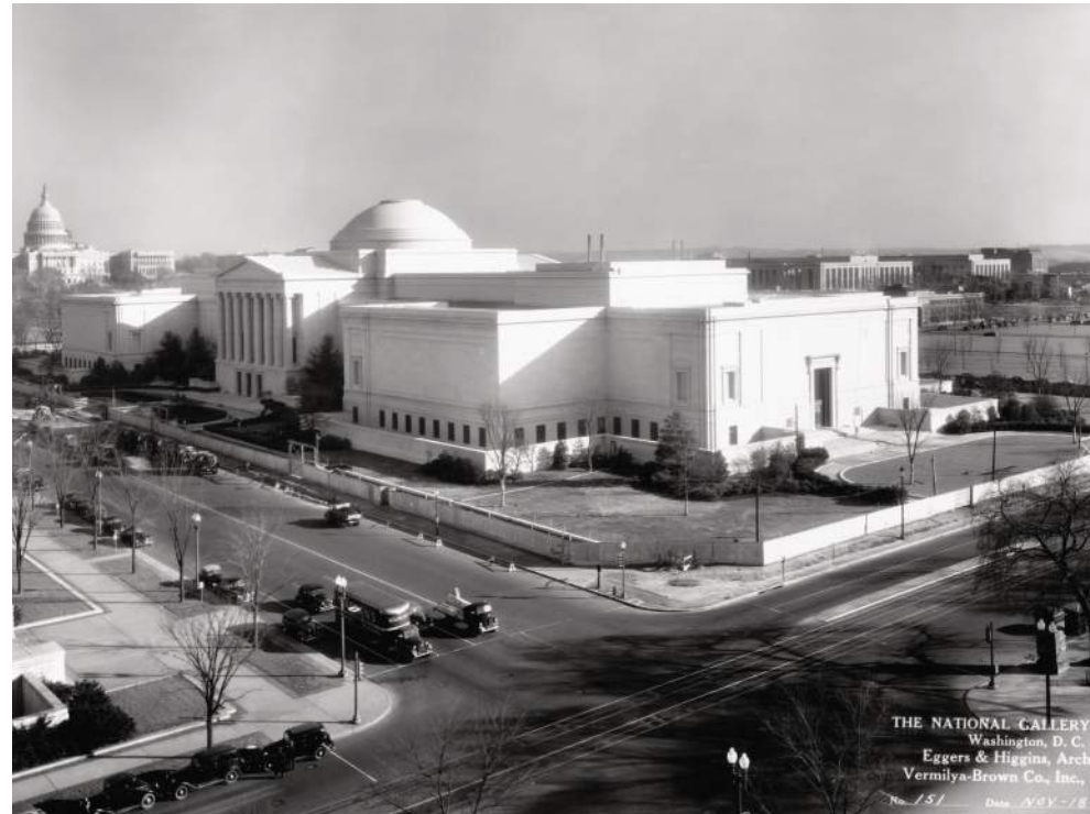
Figure 1-25. Construction progress on the West Building, November 1940. (National Gallery of Art, Washington, DC, Gallery Archives. RG26A, National Gallery of Art Architecture Images - West Building Original Construction. Photograph by Commercial Photo Co. 26A23_2289_001)
