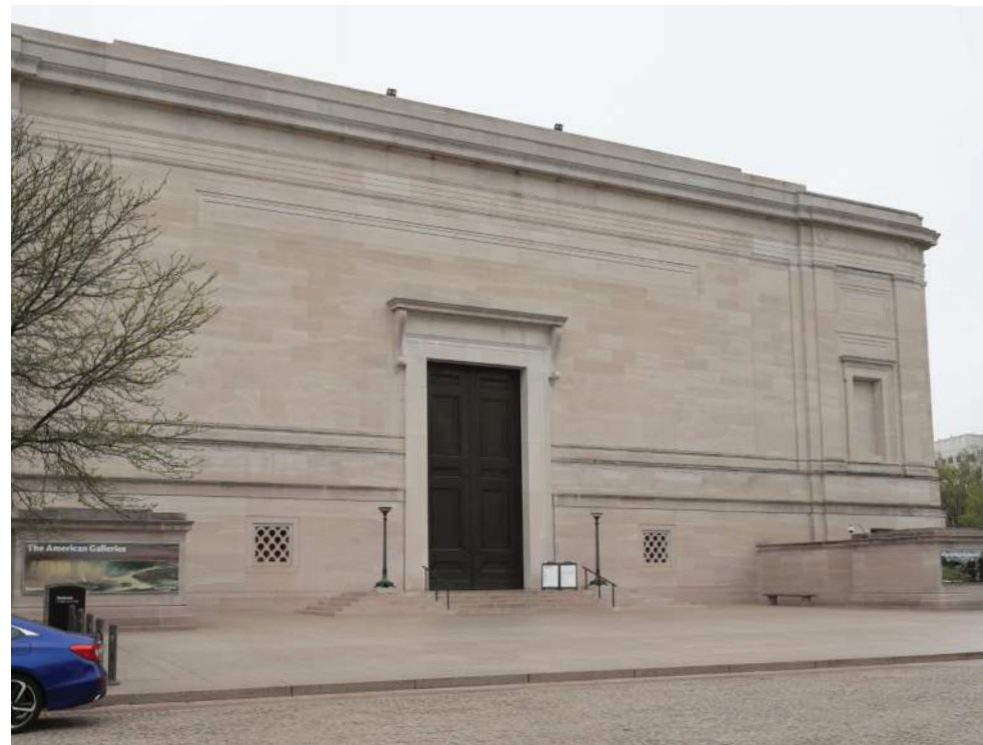
Figure 1-42. Marble landing and stairs and granite landing at the Fourth Street Entrance of the West Building.
