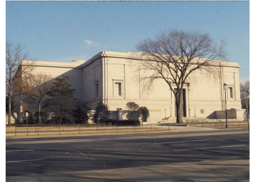
Figure 1-26. Historic photo (1971), west elevation. (National Gallery of Art, Washington, DC, Gallery Archives. RG26A, National Gallery of Art Architecture Images - Building, Campus, and Art Installation Views. 26A5_34392_004-4K)
