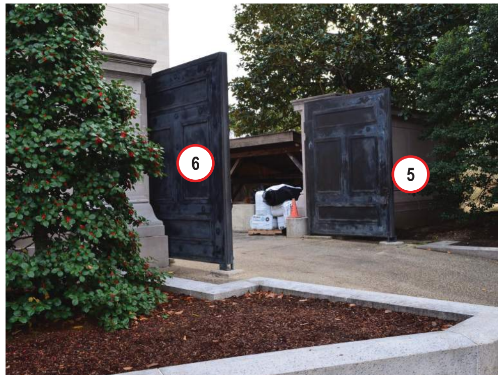
Figure 1-14. View of moat walls and open moat gates.
