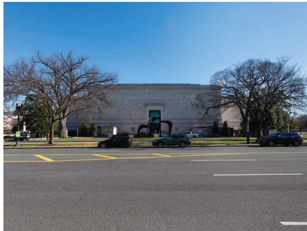
Figure 1-18. View of the Seventh Street Entrance from the entrance of the Sculpture Garden.
